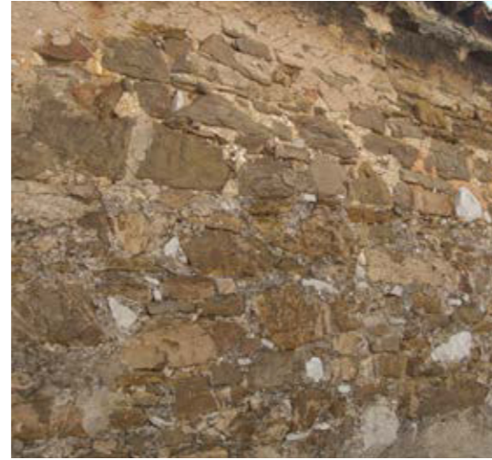
Sandstone blocks with calcite veins are irregular in shape. Occasional blocks of Alveolinid-numulitid limestone are also present (Sant' Antonio in Bosco/Boršt)
