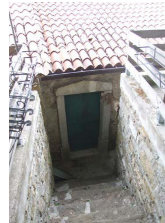
Entrance to a building from an upper terrace. The difference between elevations of nearby terraces is such that the building is entirely dug into the ground
