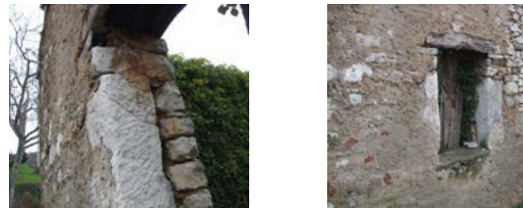
Vertical elements of the window frame (jerte) of local limestone which has been roughly surface treated, in combination with a timber lintel
