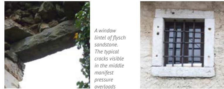
A typical window reveal of Cretaceous limestone from karst quarries
