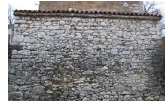
A typical outside wall showing the use of local limestone. Larger and more correctly shaped, roughly treated building stones were used for corners, while the rest of the wall comprises less correctly shaped blocks assembled in horizontal lines. Smaller rocks were used to level the surface. In between are individual blocks of flysch sandstone. They are normally smaller and used mainly for levelling the surface. The wall has traces of rough rendering and inclines to follow the terrain
