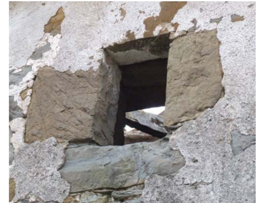
Window reveals with flysch frame
