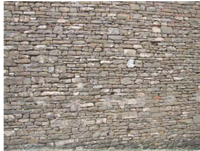
Sandstone blocks with calcite veins are irregular in shape. Occasional blocks of Alveolinid-numulitid limestone are also present (Sant' Antonio in Bosco/Boršt)
