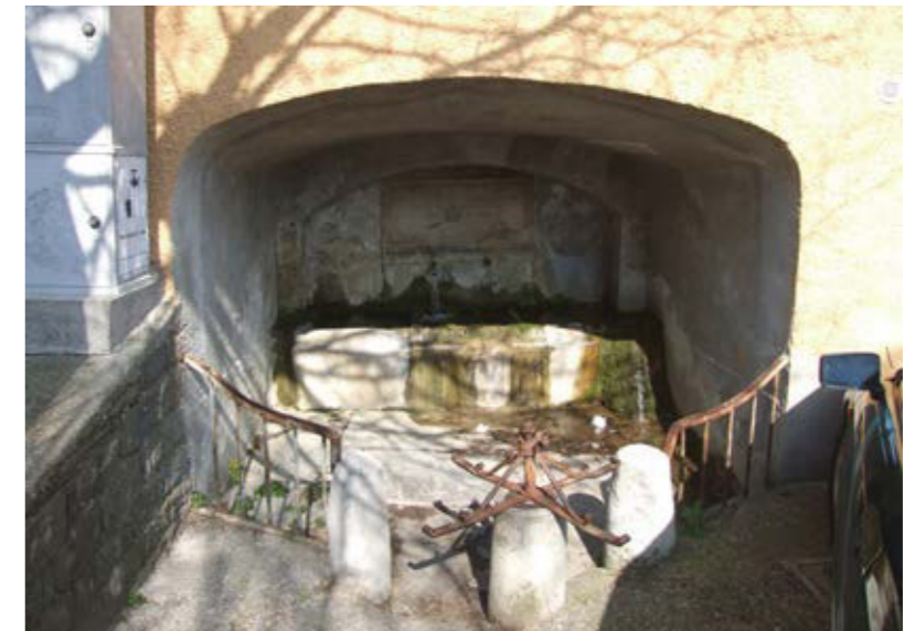
A public well in the village of Sant' Antonio in Bosco/Boršt. The bollards and inscription plate are fashioned from Alveolinid-numulitid limestone
