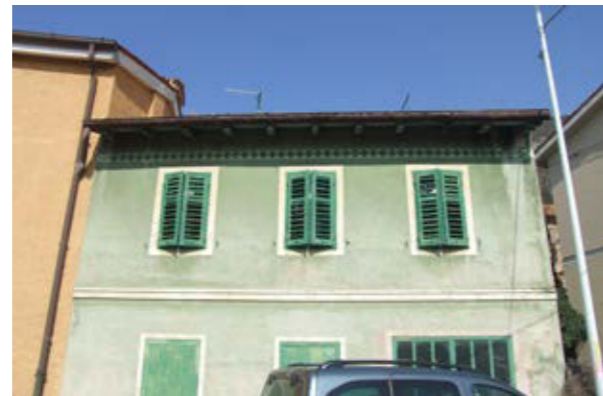
An ornamented extended overhang and shutters with movable elements show a bourgeois influence in this construction
