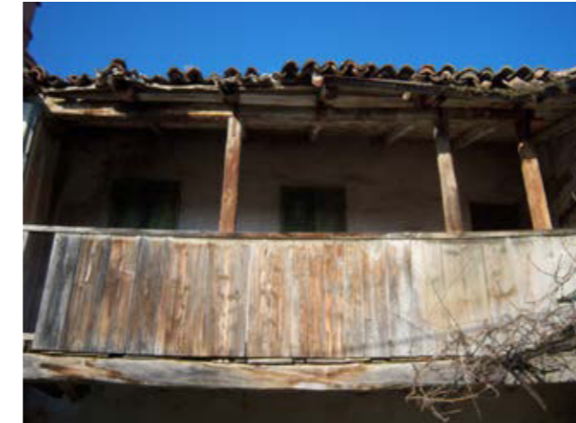
A timber balcony
