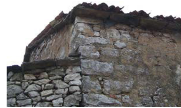
An eave of flysch sandstone grooved roofing tiles and a gabled wall with a row of flysch sandstone grooved roofing flags
