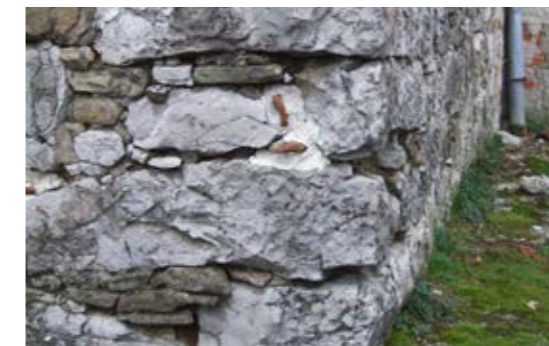
Roughly treated corner stones from alveolina nummulitic limestone
