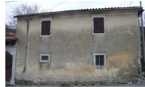
A short semicircular plastered eave over a timber subframe
