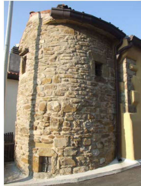
A wall with sandstone pebbles in Bagnoli della Rosandra/Boljunec
