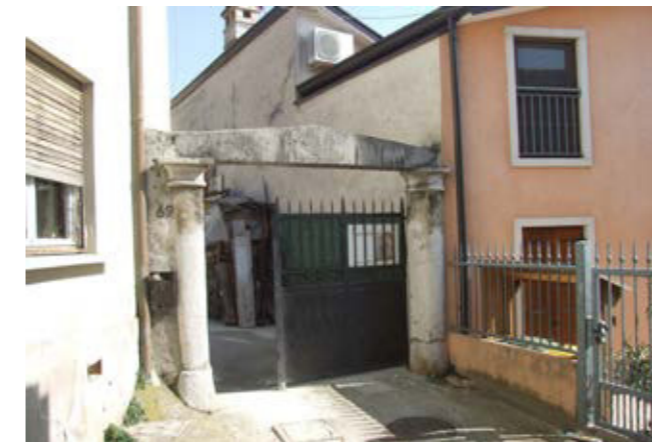
Architrave made of sandstone from the Transitional Beds of Sant' Antonio in Bosco/Boršt
