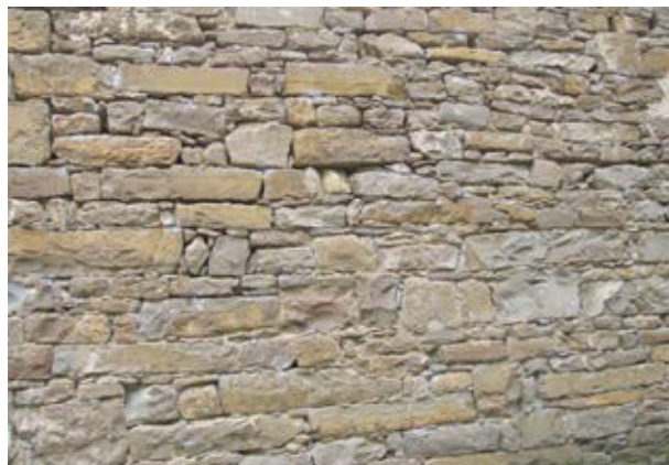
Characteristic construction of peripheral walls from flysch sandstone
