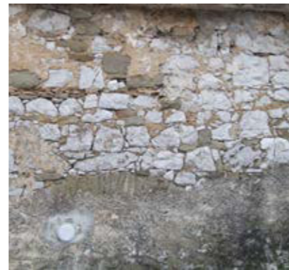
Remains of an immured arch of flysch sandstone building blocks
