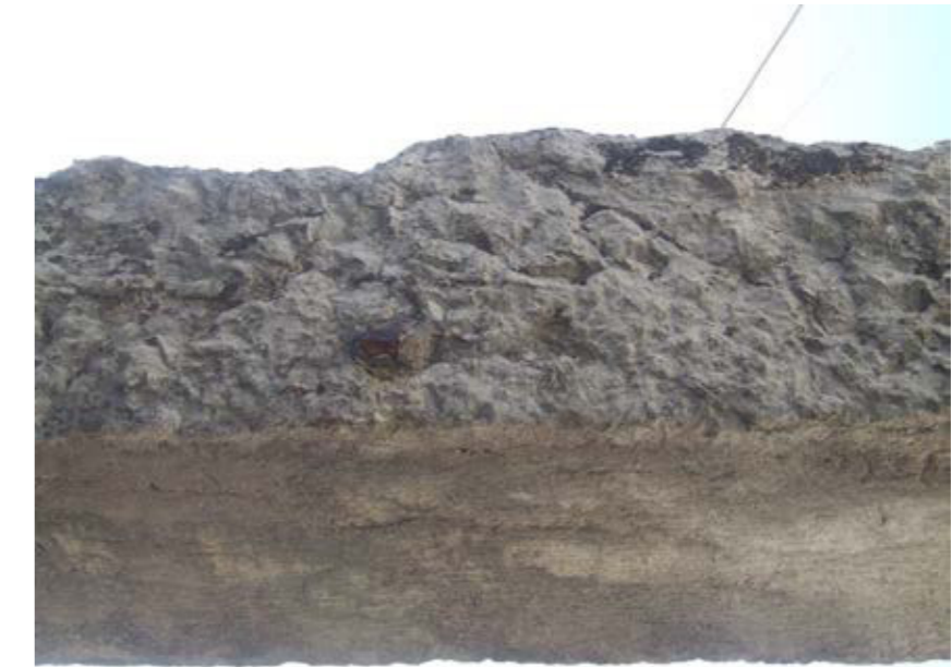
A detail of the rear side of the Architrave reveals it was originally built-in, and appears here in secondary use
