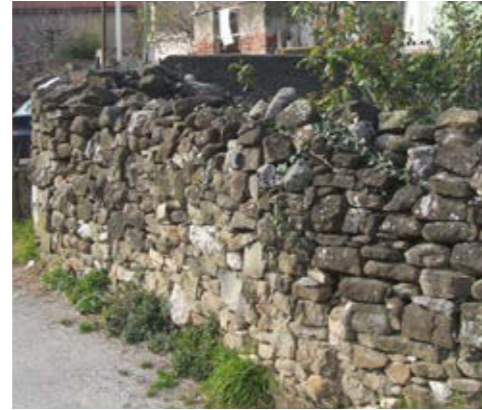
A wall with sandstone pebbles in Bagnoli della Rosandra/Boljunec
