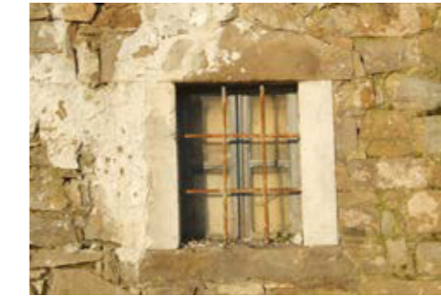
A window frame which reuses side pylons of cretaceous limestone taken from another building
