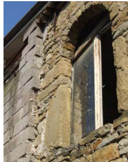
A window reveal with a frame and arch of flysch sandstone
