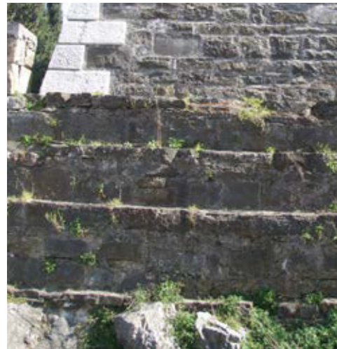
Dolina is built on large limestone (and breccia) boulders
