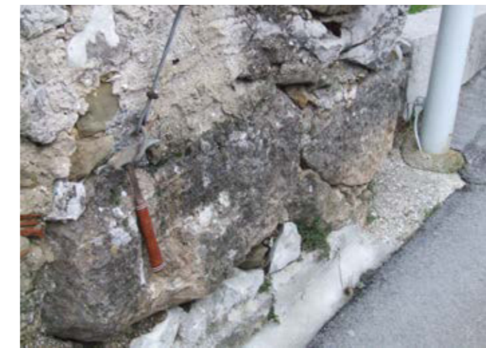
Two larger flowstone building blocks. Judging by their treatment, they probably came from nearby caves which are numerous in this area
