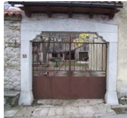
A1 Grozzana/Gročana House No33 A stone portal with a pointed lintel, hewn capitals and bases of Cretaceous limestone. The latter was mainly brought from karst quarries, which is also reflected in architectural elements typical of karst quarrying in the second half of the 19th Century. The canopy above the portal offers weather protection
