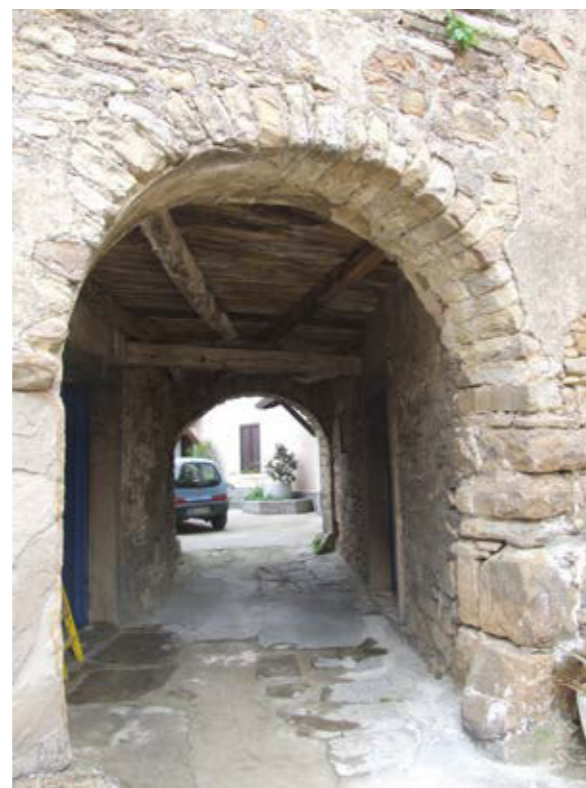
A view of a flysch sandstone portal offering access to a kort
