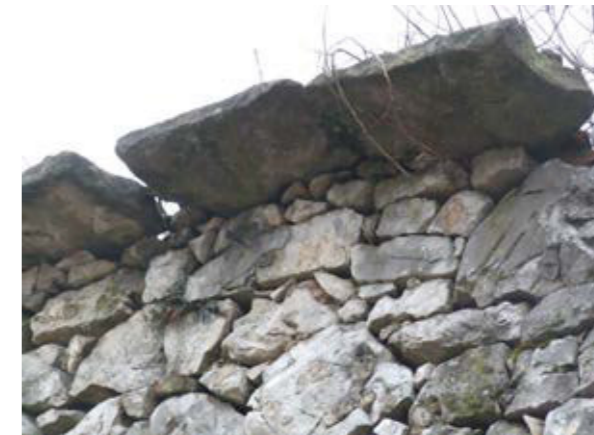
B3 An eave of limestone grooved roofing flags
