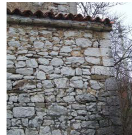
B2 An eave of flysch sandstone grooved roofing flags
