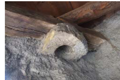
A stone hook used to fasten the door spindle
