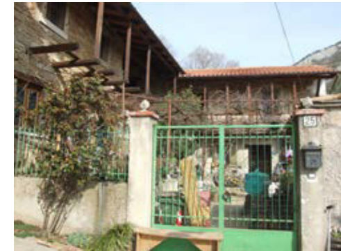
Timber console balconies
