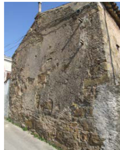
The size of these building blocks is not characteristic of traditional construction
