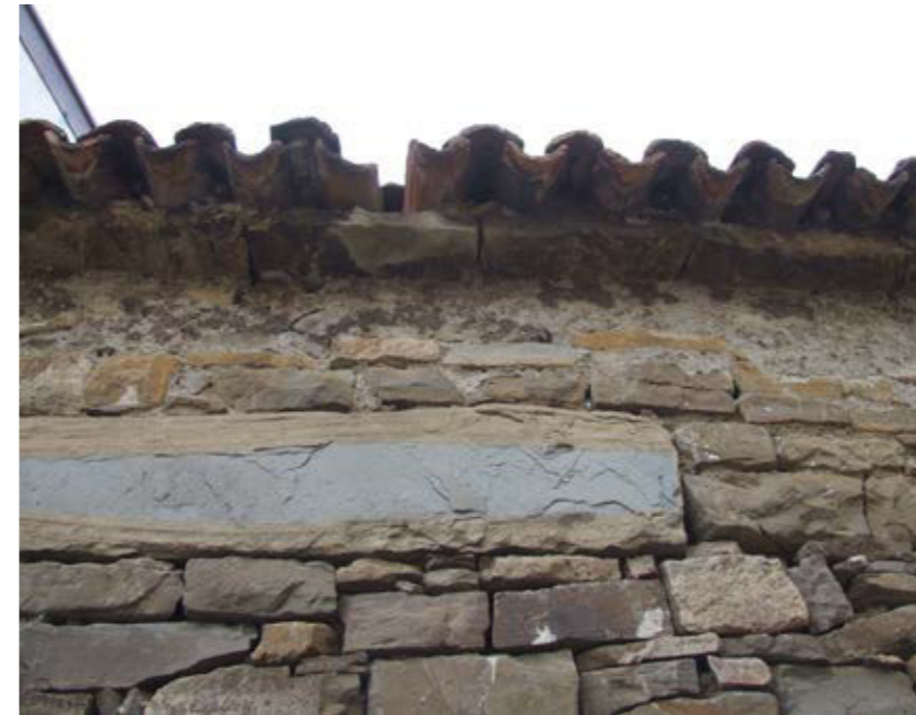
A partly-weathered block of flysch sandstone with lamination in the upper part (Prebenico/Prebeneg)
