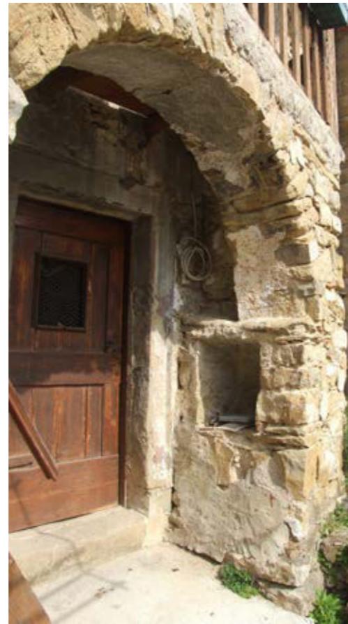
A view of the construction of the arched element
