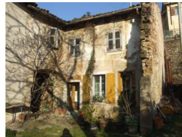
An outside area and the structure of a wall
