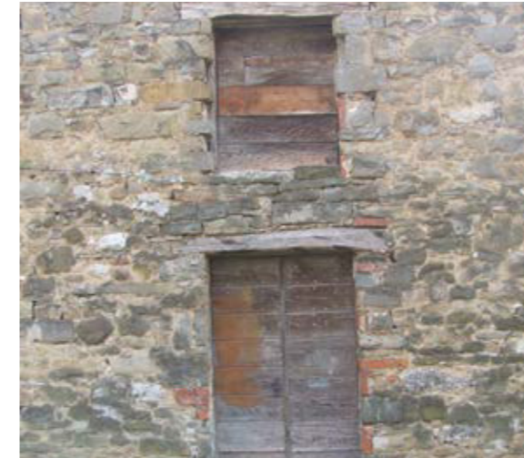
Blocks of slope breccia and flysch sandstone pebbles in a wall in Bagnoli della Rosandra/Boljunec
