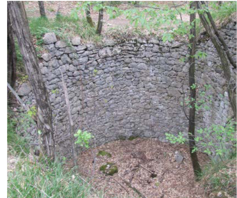
The use of roughly-shaped stone blocks for construction of ice storage sheds between Pesek and Draga villages
