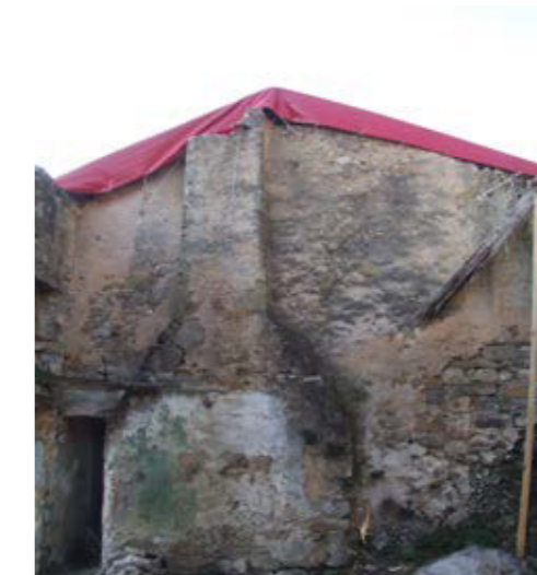
An outward projecting fireplace
