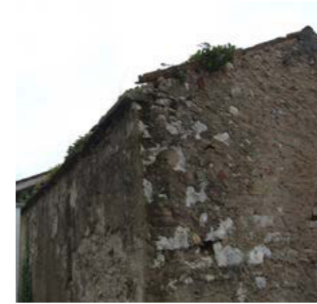
B1 An outbuilding at House No 20 in Grozzana/Gročana A stone plate eave of flysch sandstone A side wall without an eave featuring a row of grooved roof tiles in line with the façade
