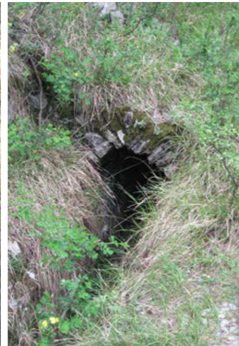
A vault of the Roman aqueduct made from Alveolinid-numulitid limestone and flysch sandstone (left), and of Alveolinid-numulitid limestone exclusively (right)
