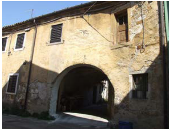
An arched underpass offers access to the shared area behind a row buildings
