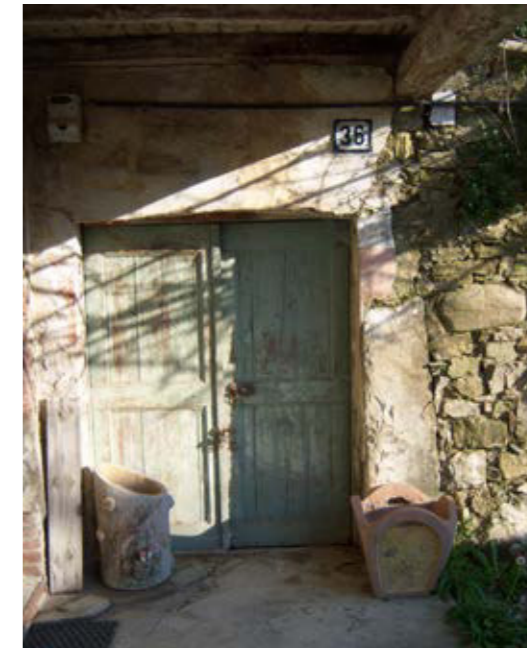
A gate reveal of flysch sandstone which was entirely rendered
