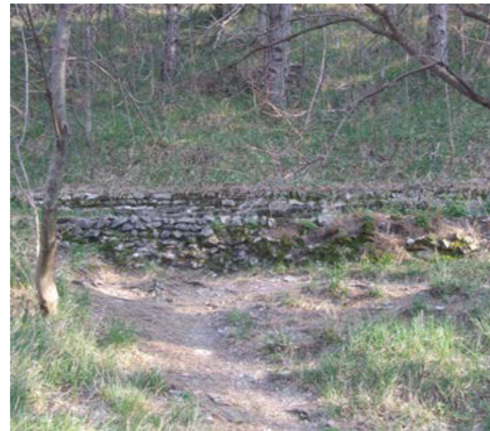
Aqueduct channel made of local Alveolinid-numulitid limestone
