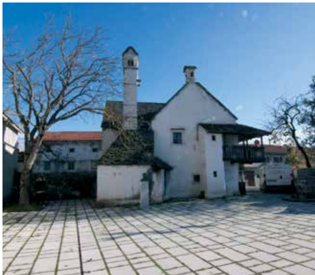
Figure 10. New stone paving made of platy limestone. Elements are cut into regular shapes, grouts are open with grass growing in them. The square provides for good drainage of rainwater. With its clear modular orthogonal network and different sizes of stone, it creates a dynamic surface in the inner courtyard. Divača, Slovenia.
