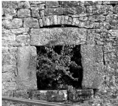
Figure 8. Loading and the reason for the distribution of openings along the axis of the building shell. A small pressure-relief arch above a stone lintel distributes the vertical load to the edges of the opening.
