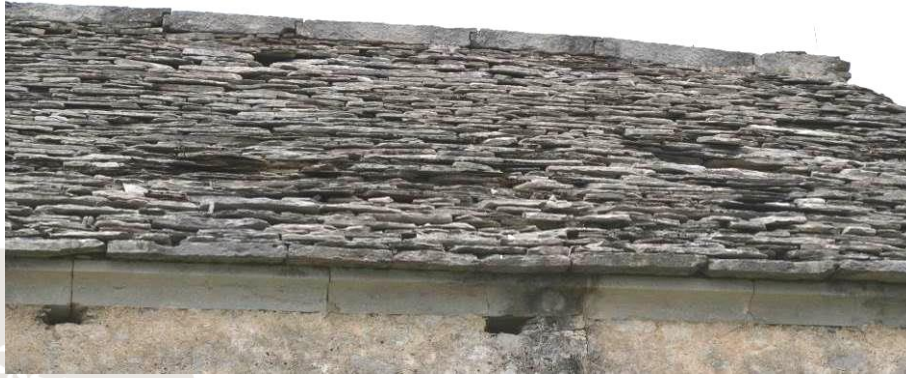
Figure 3.13 A detail from the roof of the church on Gura hill. The platy limestone of Povir Fm. (dark fields) is disintegrating due to its lower-quality. Fractured Repen limestone (~ 70% of the roof) is more resistant to external atmospheric conditions.
