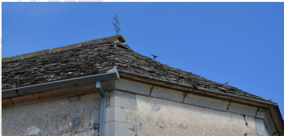
Figure 5.10 The church in Kopriva roofed by Komen limestone from the Sežana Fm.
