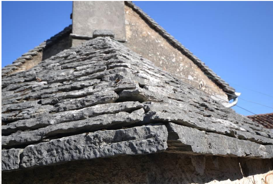
Figure 5.15 The use of fractured Repen limestone for roofing in Gorenje pri Divači (southern Kras, Slovenia)
