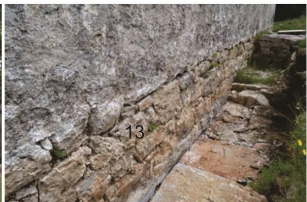
Parts of the building (elements): 1-walls, 13-church foundation
