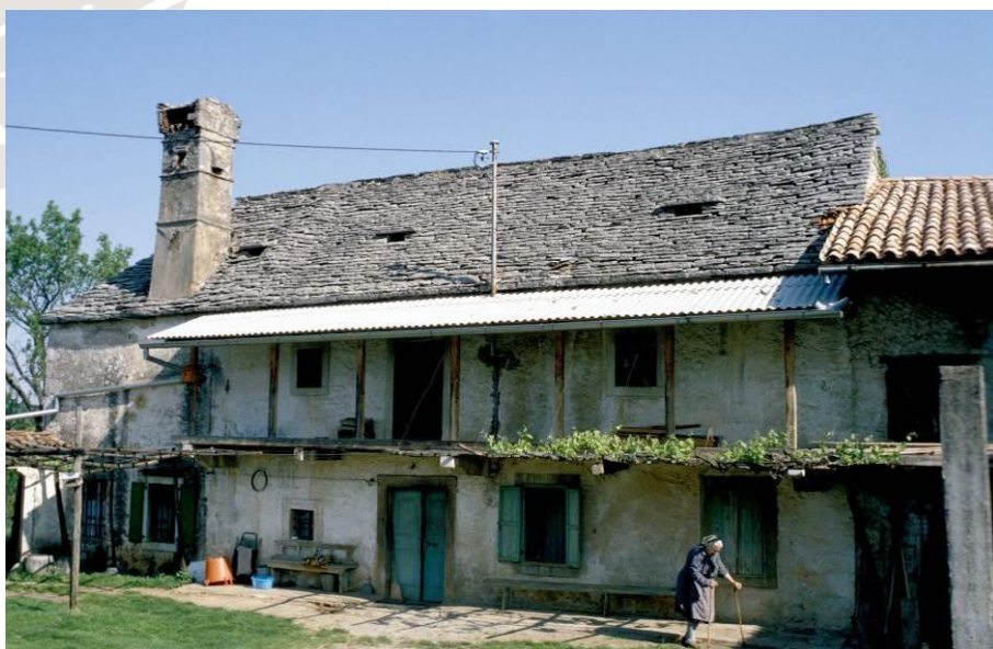
Figure 5.13 Rural house in Kazlje roofed using Tomaj limestone (archive photo, B. Jurkovšek).
