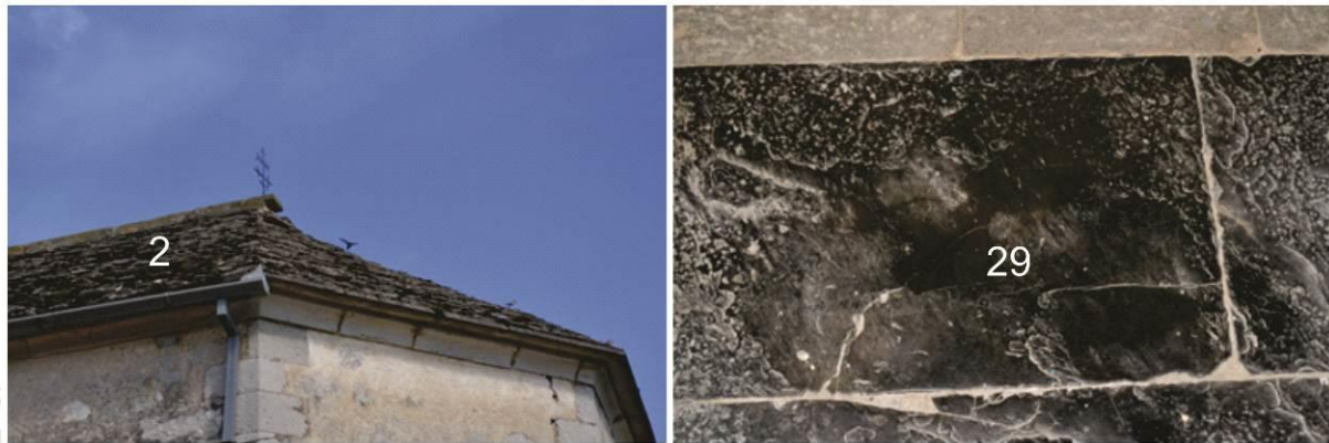
Parts of the building (elements): 2-roof, 29-vestry floor
