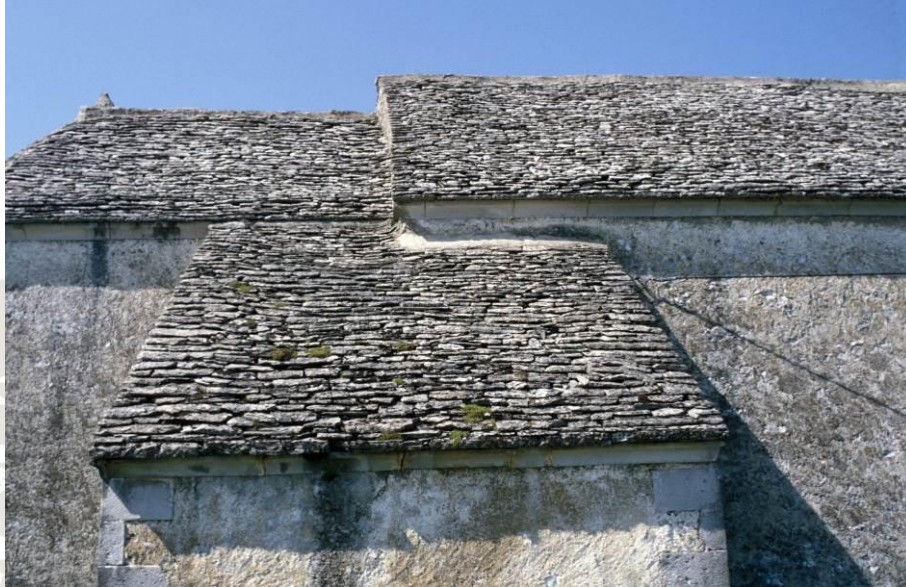
Figure 5.14 The church in Križ was originally roofed using Tomaj limestone (archive photo, B. Jurkovšek).
