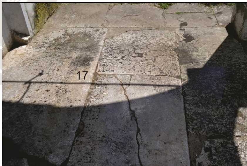
Part of the building (element): 17-entrance shed floor
