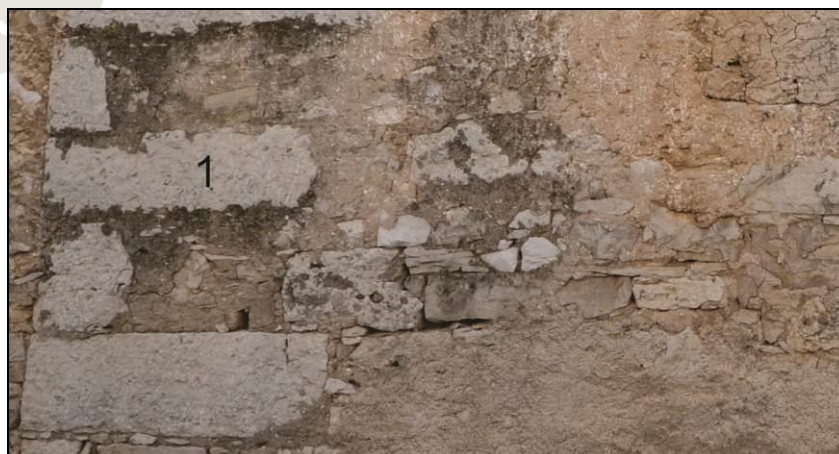
Part of the building (element): 1-walls
