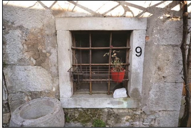
Part of the building (element): 9-window frame (kitchen)
