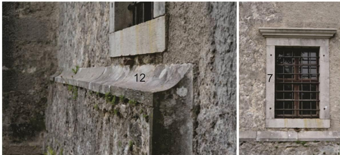
Parts of the building (elements): 7-window frames (three on the church south wall), 12-final stone
