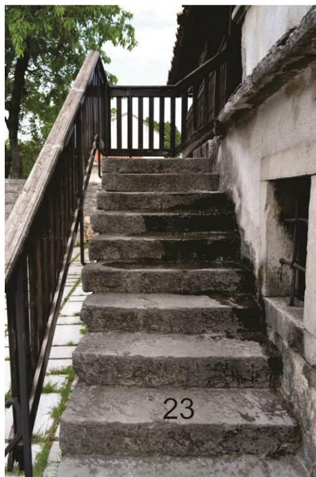
Part of the building (element): 23-stairs
