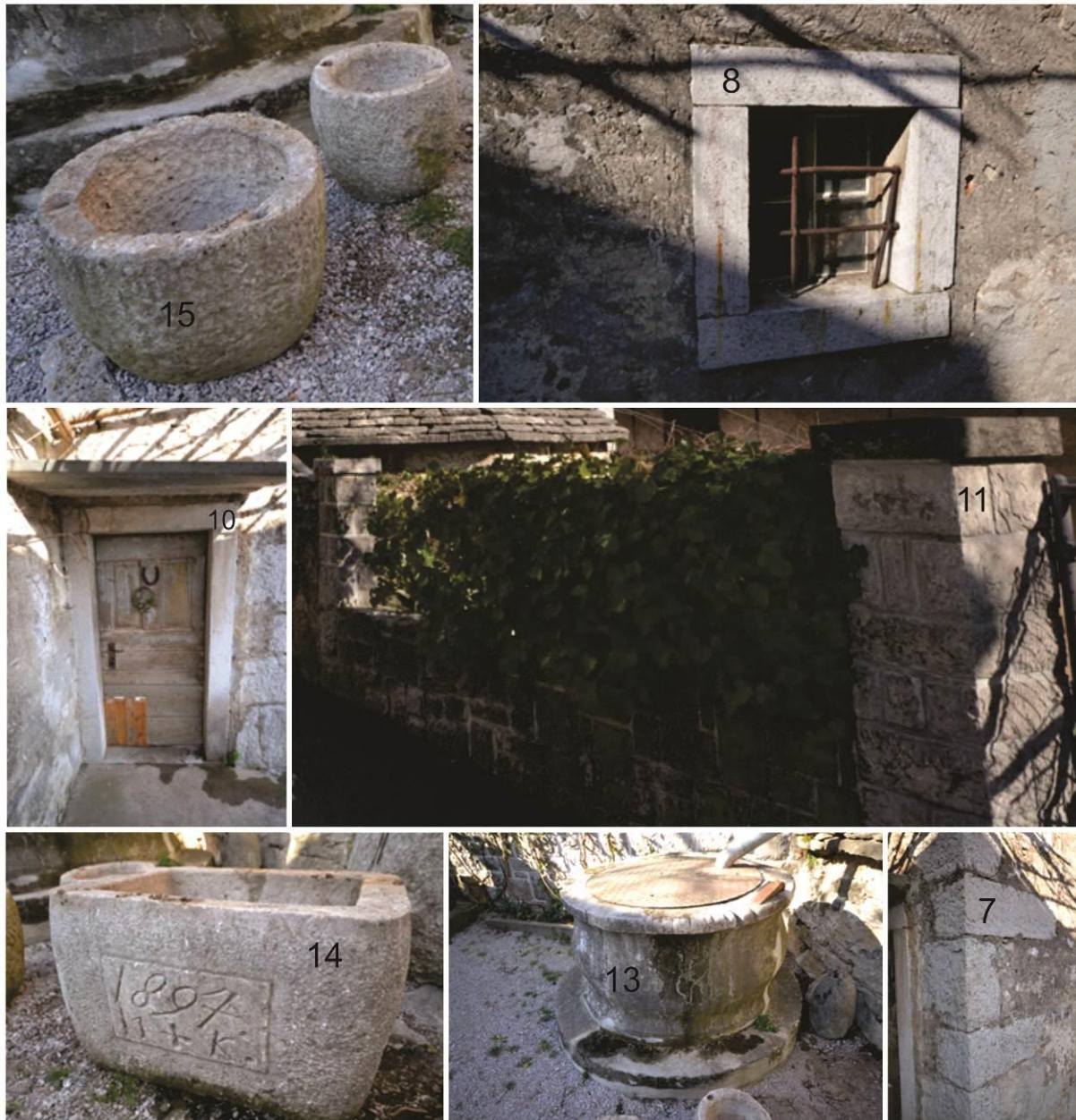
Parts of the building (elements): 7-corner stones, 8-window frame, 10-doorpost, 13-cistern rim, 14-trough, 15-stone vessel
