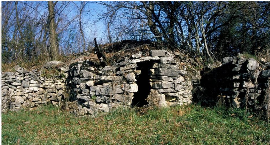
Figure 5.4 Field-shelter partly built of Komen platy limestone from the Povir Fm. near Volčji Grad village.
