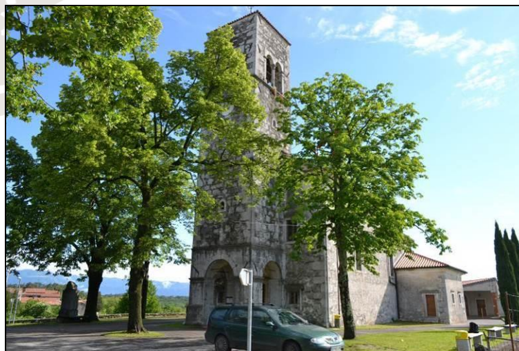
Figure 3.6 Church in Kopriva, view from the west.
