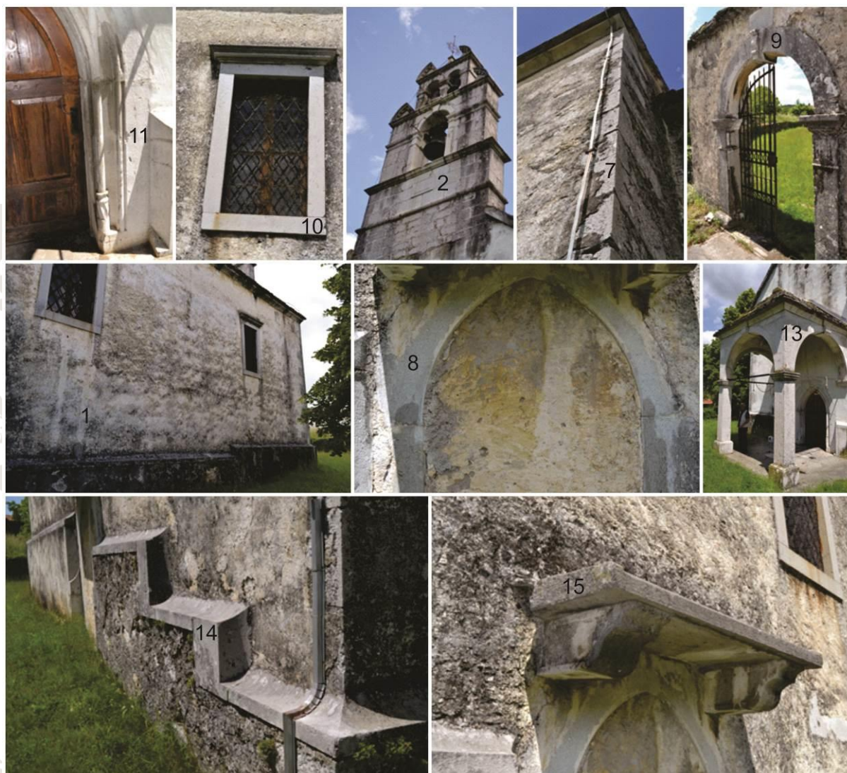
Parts of the object (elements): 1-walls, 2-bell tower walls, 7-corner stones, 8-former entrance doorpost, 9-external entrance doorpost, 10-window frames, 11-main doorpost, 13-entrance shed corbels, 14-final stone, 15-former shed entrance and brackets
