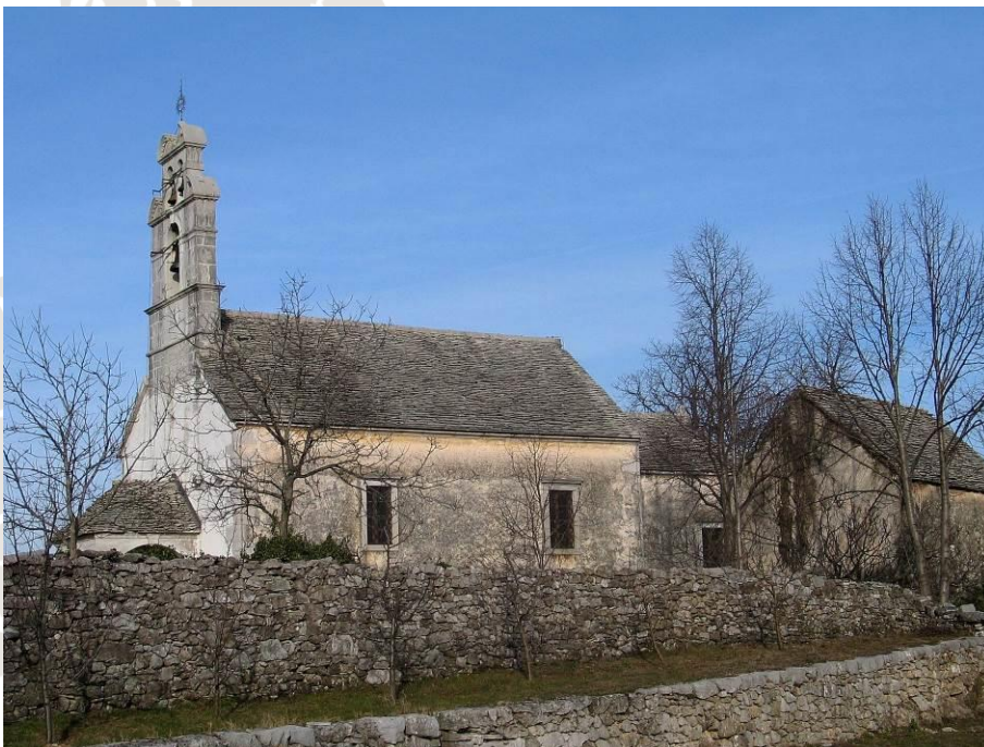
Figure 5.6 The church in Šmarje pri Sežani roofed by Komen limestone from the Povir Fm.
