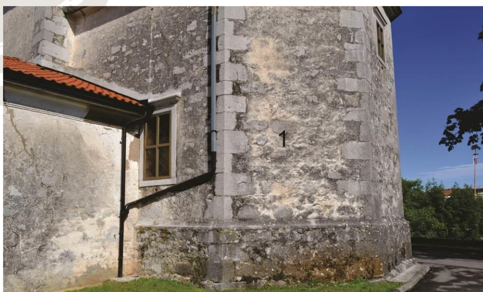
Part of the building (element): 0-walls, general
