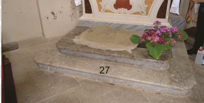
Part of the building (element): 16-left side-altar stairs
