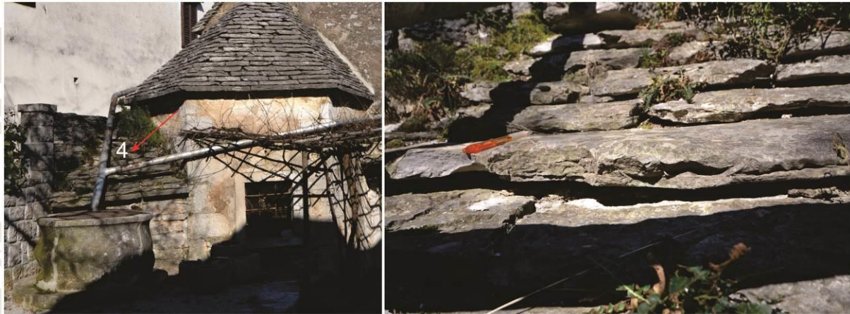
Part of the building (element): 4-oven roof
