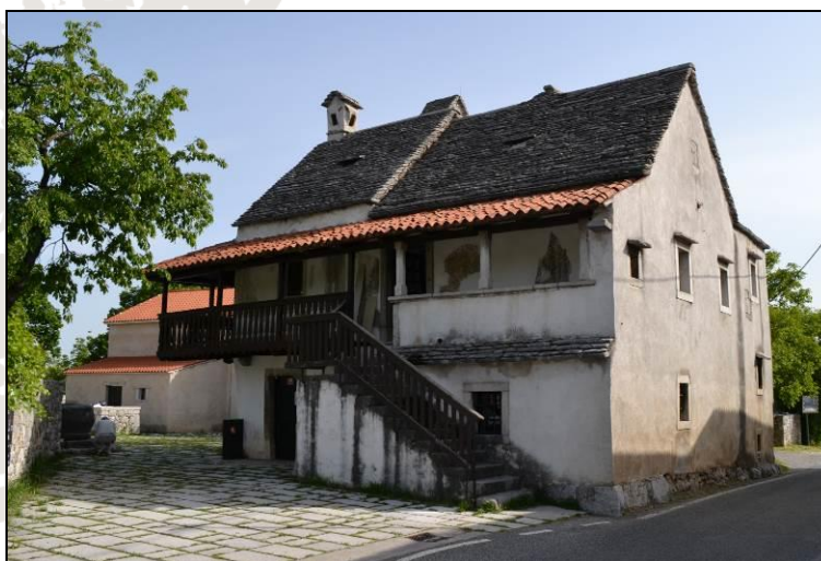
Figure 3.3 Škrateljnova homestead, view from the south
