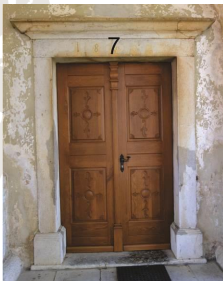
Part of the object (element): 7-main entrance doorpost
