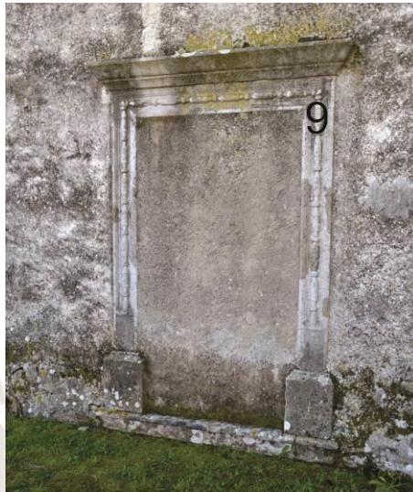
Part of the object (element): 9-former entrance doorpost
