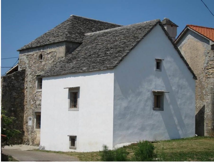
Figure 5.5 A recently renovated house in Gabrovica, roofed with Komen platy limestone from the Povir Fm. from the close vicinity of the village.
