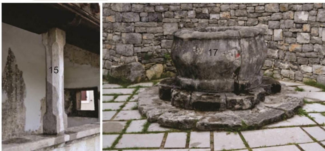
Parts of the building (elements): 15-middle balcony column, 17-cistern
