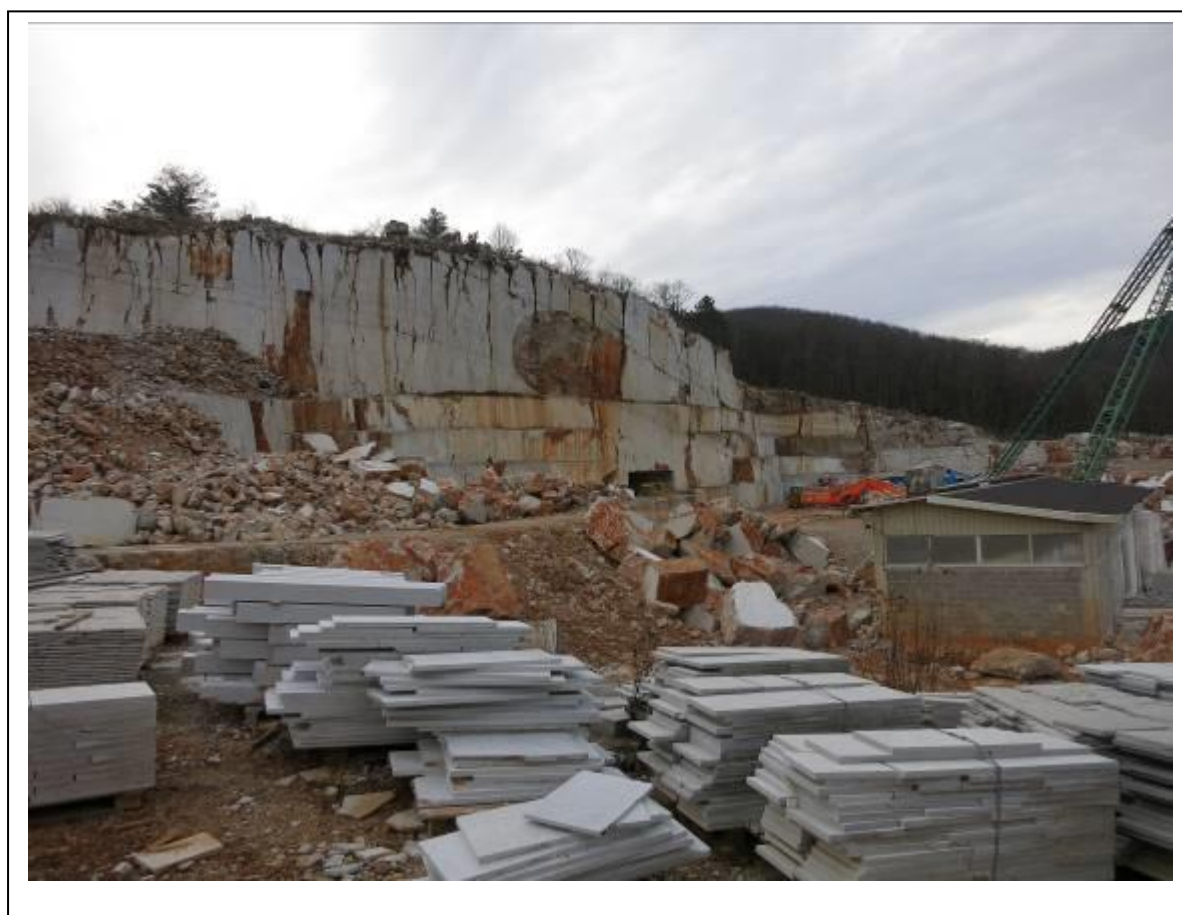
Photo IIIA -1: Debela Griža (Tavčar quarry). At the back wall of the quarry, the fractured limestone is clearly visible.
