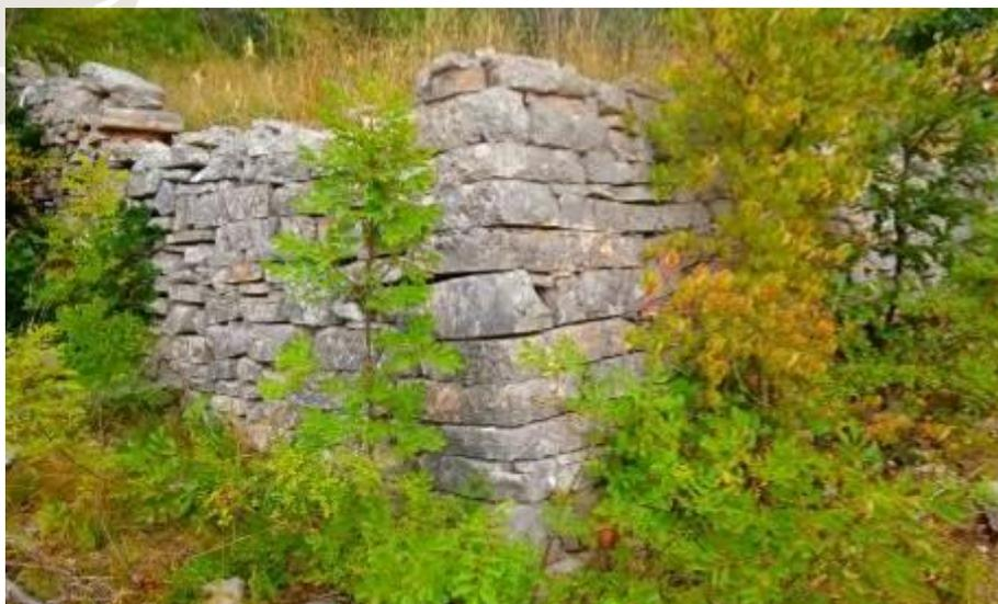
Figure 4.31. Old dry-walls built of Boričevac Lower Paleogene platy limestones.
