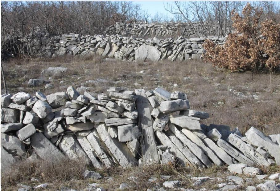
Fig 4.8. Interesting and picturesque old dry walls made of Podveležje platy limestone north of the village of Podveležje.
