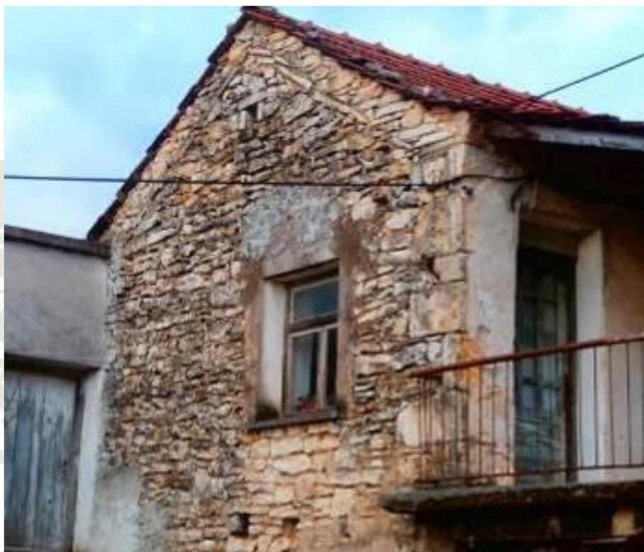
Figure 3.31. One of many older houses with walls made of platy limestone from the Miocene age, at Široki Brijeg.
