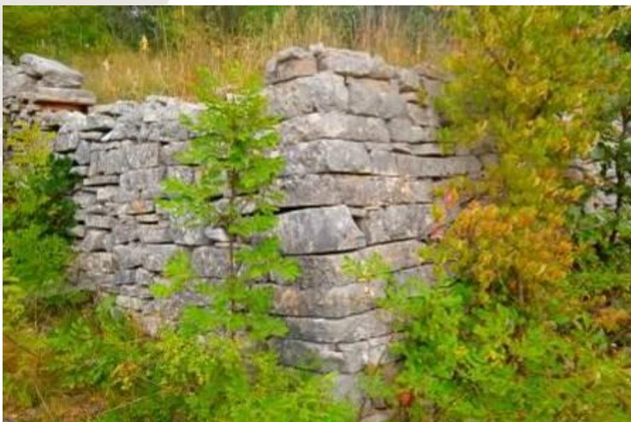
Figure 3.30. Impressive old dry wall, made entirely of platy limestone from the Paleocene age, on the Boričevac site.
