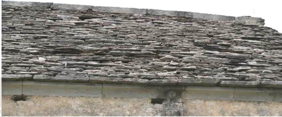
Figure 3.13 A detail from the roof of the church on Gura hill. The platy limestone of Povir Fm. (dark fields) is disintegrating due to its lower-quality. Fractured Repen limestone ( ~ 70% of the roof) is more resistant to external atmospheric conditions.
