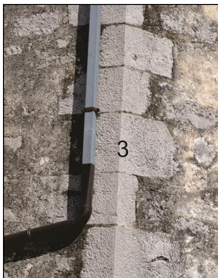
Part of the building (element): 3-corner stones
