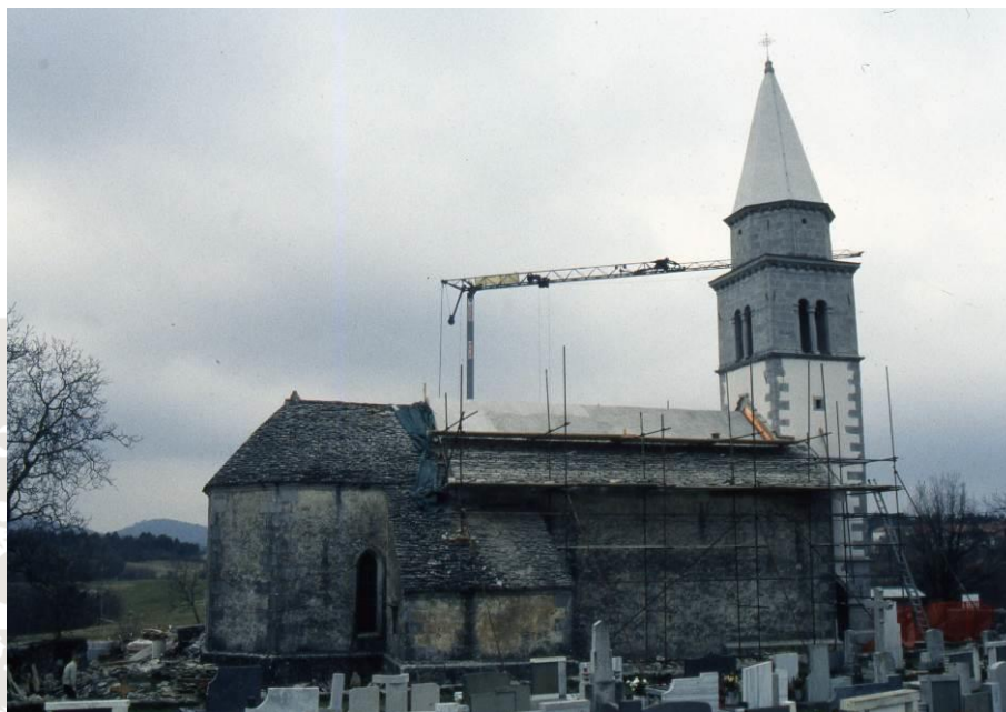
Figure 5.17 Renovation of the roof on the church in Križ village. Originally it was roofed using Tomaj limestone, which was partly replaced by the fractured limestone from the Lipica Fm. (archive photo, B. Jurkovšek).
