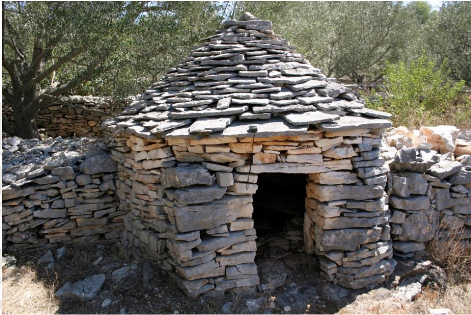
Figure 19: Case of roof structure without additional roof supporting structure. Corbelling is building technique used for simple stone structures as hiška, kažun, vrtujak and other structures in this area. Vrtujak, Korčula, Croatia. Photo: Domen Zupančič.
