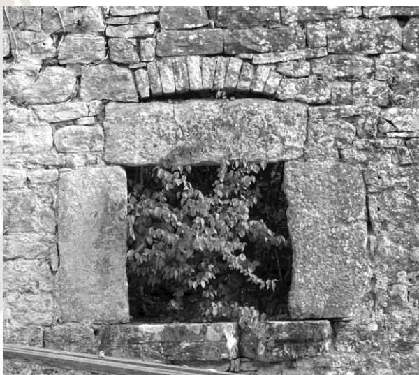
Figure 25: Explanation of weight repositioning combined with wall openings. Small arch redirects the weight of the wall to the sides of the opening.
