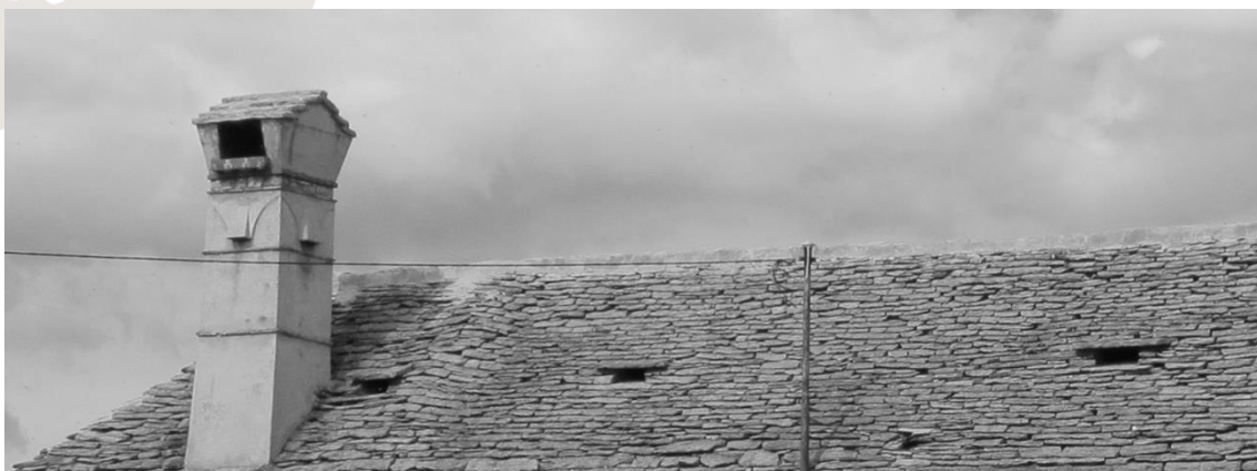
Figure 5: Stone roof and roof openings, Kazlje, Slovenija. Source: Neža Čebtron.
