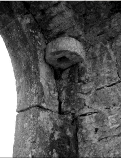
Figure 37: Driving stone for entrance door axis.
