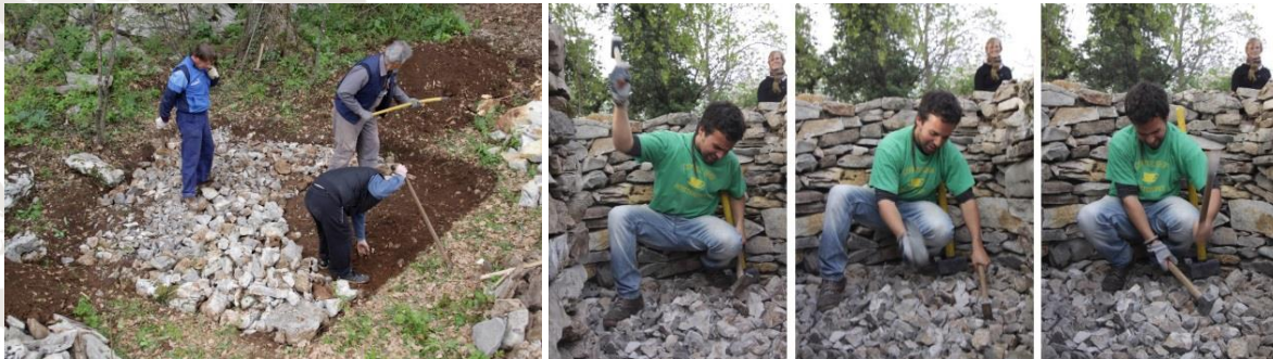
Figure 42: Stone base flooring and its finalization at stone shelter in Slovenia. It is used only rest of stone of platy limestone plates. Photo: Domen Zupančič.
