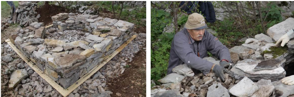
Figure 3: Photos of construction of hiska at Lipica, Slovenia, 2012. Source: Domen Zupančič.
