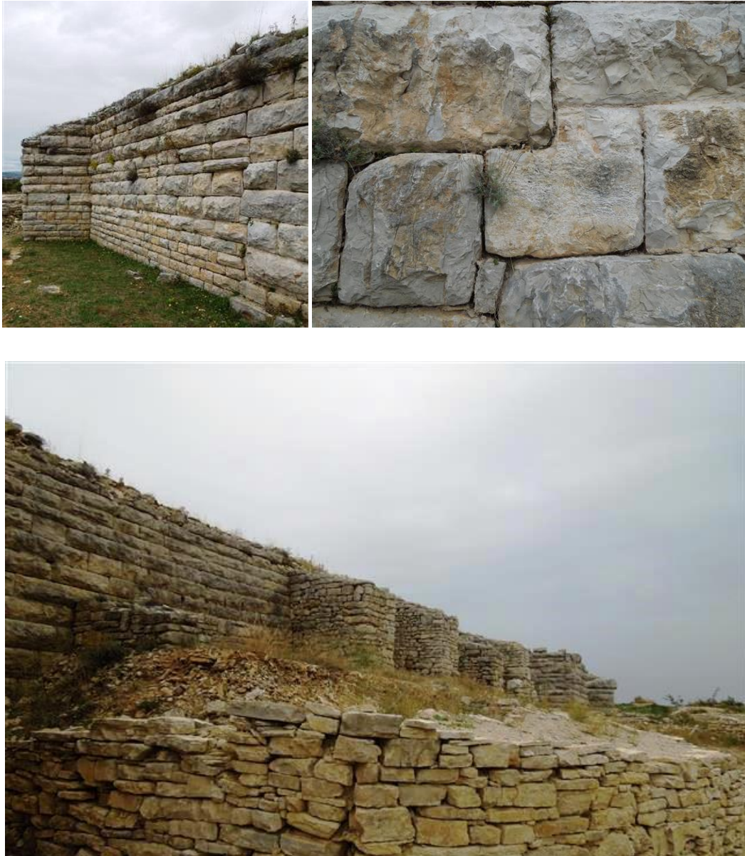
Figure 3 Roman Asseria , built of platy limestone (CRO). A fine example of the limestone layers of different thickness.
