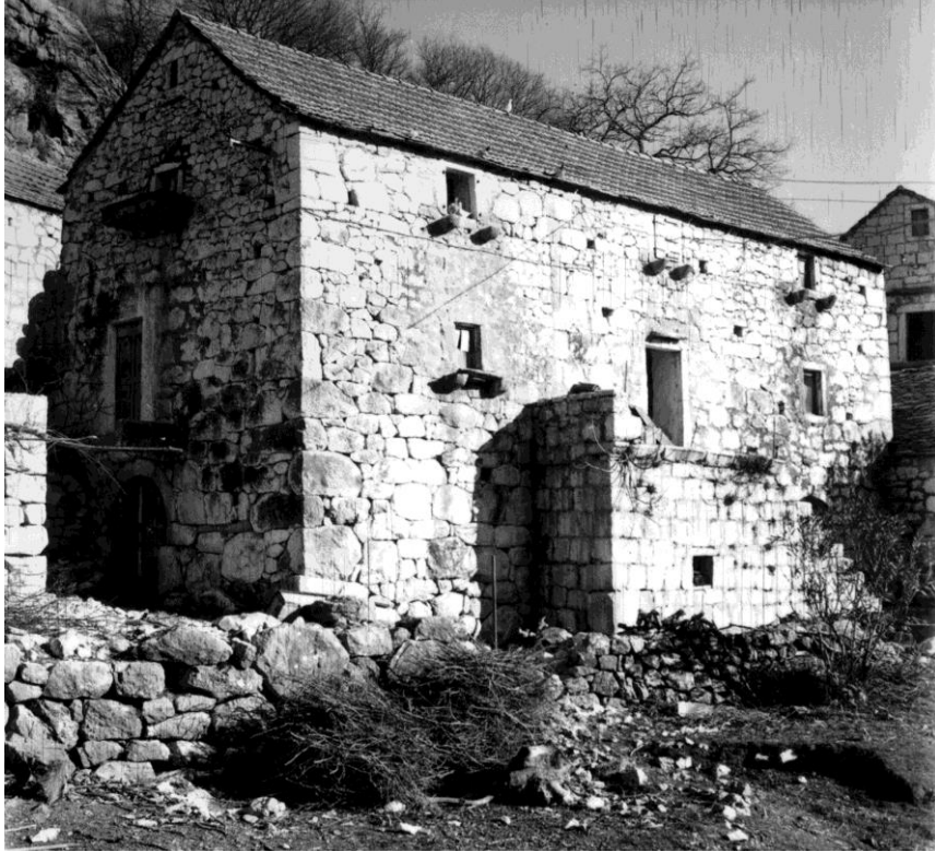
Stone walls of the house of Mile Gojsalić, Kostanje. Dry wall and semi-carved stone with lime mortar.
