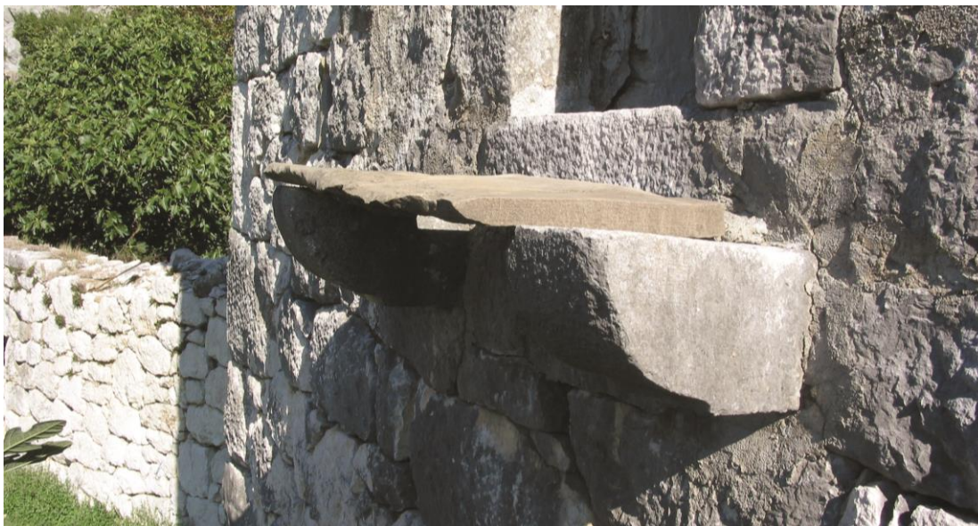
Kostanje, the Gojsalić complex, stone slabs on consoles under the window
