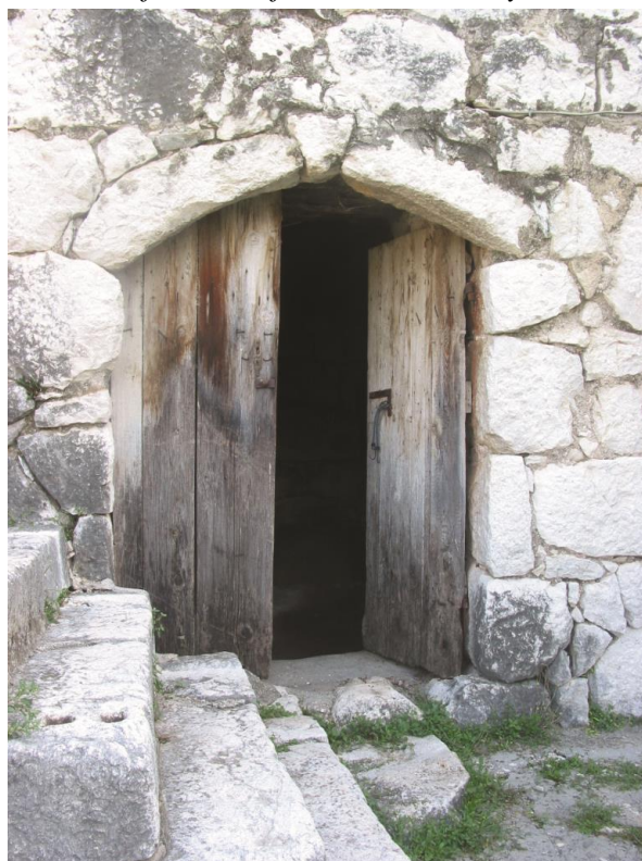
Kostanje, the Gojsalić complex, three-part arch above the door
