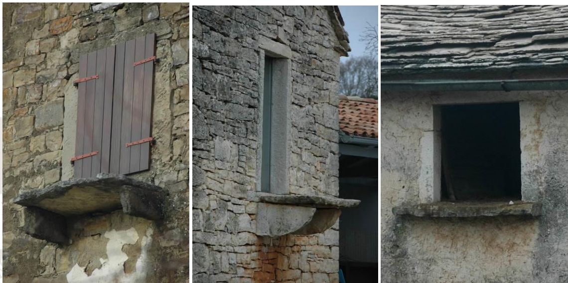
Picture 21, 22,23. Window shelf in Pirelići, window shelf with corbels made with stone slates in Radetići and a stone shelf incorporated in a window in Badnjevari.
