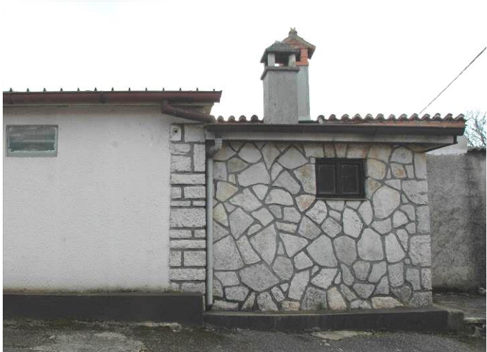
Pictures 3 and 4. Examples of bad practice in using stone slates for decorative purposes (south Istria)
