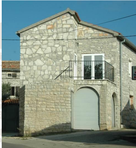
Pictures 3 and 4. Examples of bad practice in using stone slates for decorative purposes (south Istria)
