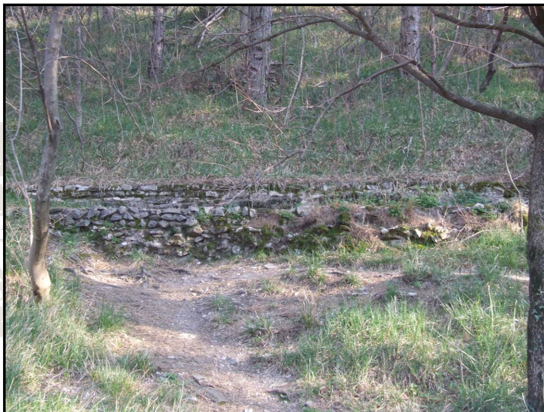
Figure 18. Aqueduct channel made of local Alveolinid-numulitid limestone.
