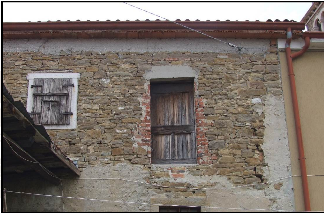
Figure 54. A wide range of building block sizes and above all, thin building blocks, are likely indicators of local sourcing (Prebenicco-Prebeneg).
