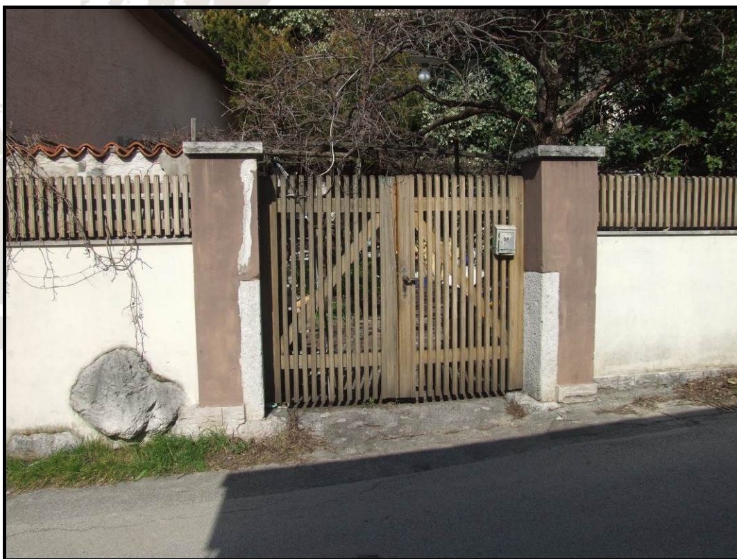
Figure 51. A large boulder from the rockfall was incorporated into the wall in situ .
