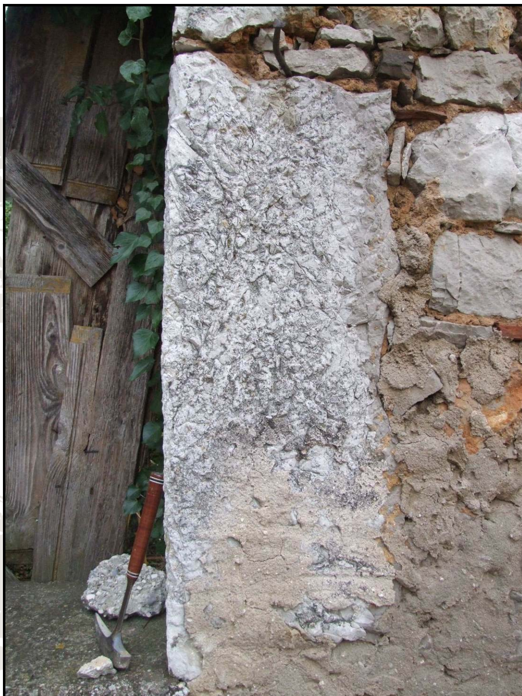
Figure 12. A poor quality stone frame made from local Alveolinid-numulitid limestone (Grozzana-Gročana).
