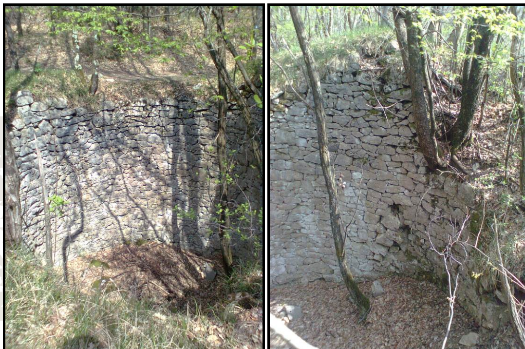
Figures 13 (left) and 14 (right). The use of roughly-shaped stone blocks for construction of ice storage sheds between Pese-Pesek and Draga villages.
