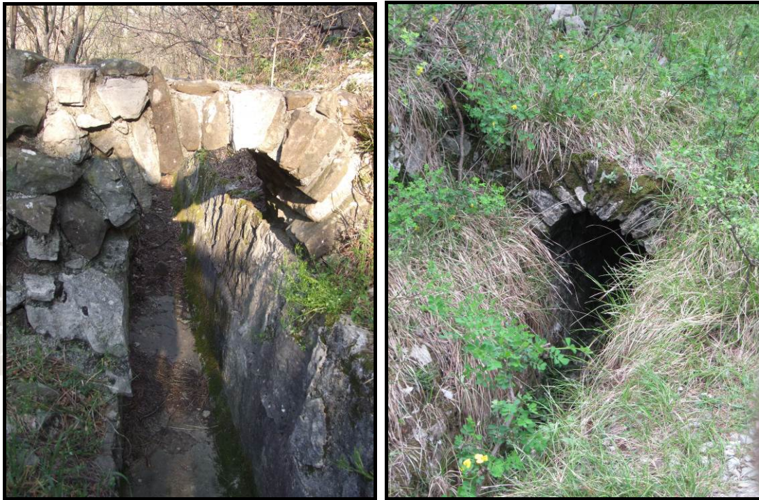
Figures 16 and 17. A vault of the Roman aqueduct made from Alveolinid-numulitid limestone and flysch sandstone (left), and of Alveolinid-numulitid limestone exclusively (right).
