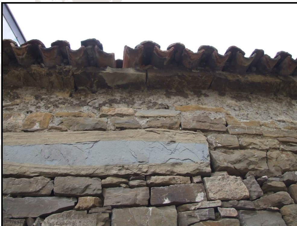
Figure 27. A partly-weathered block of flysch sandstone with lamination in the upper part (Caressana-Mačkolje).
