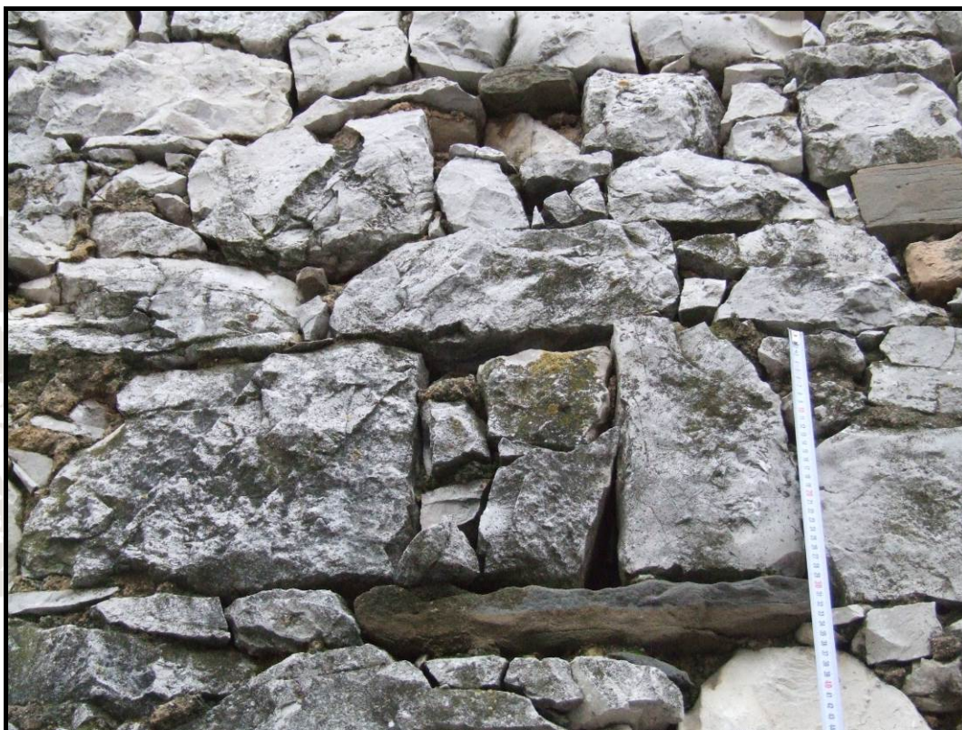
Figure 46. Roughly shaped building blocks made from local limestone used for portholes.
