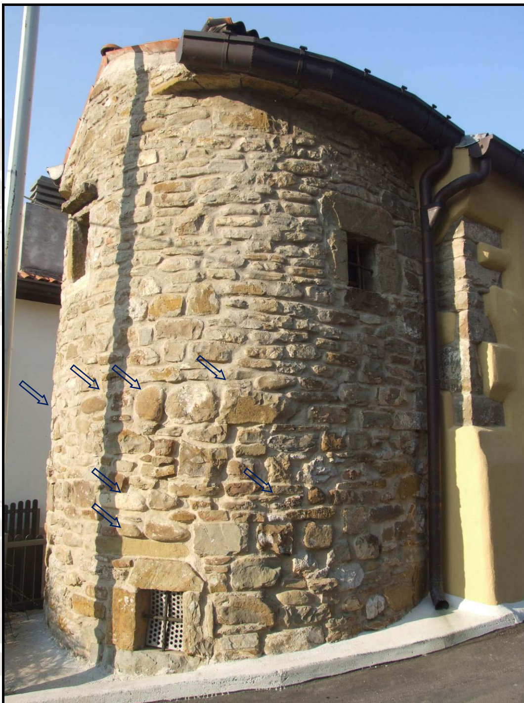
Figure 37. Large flysch sandstone pebbles in a building in Bagnoli-Boljunec.
