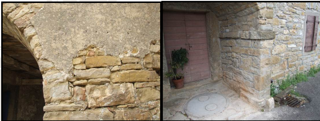
Figures 55 and 56. The poor quality of the flysch sandstone building blocks (lamination) and large variations in block sizes are common in older buildings (left); better materials in some other buildings (right) at Caresana-Mačkolje indicates the same pattern of acquiring building materials as in other villages.
