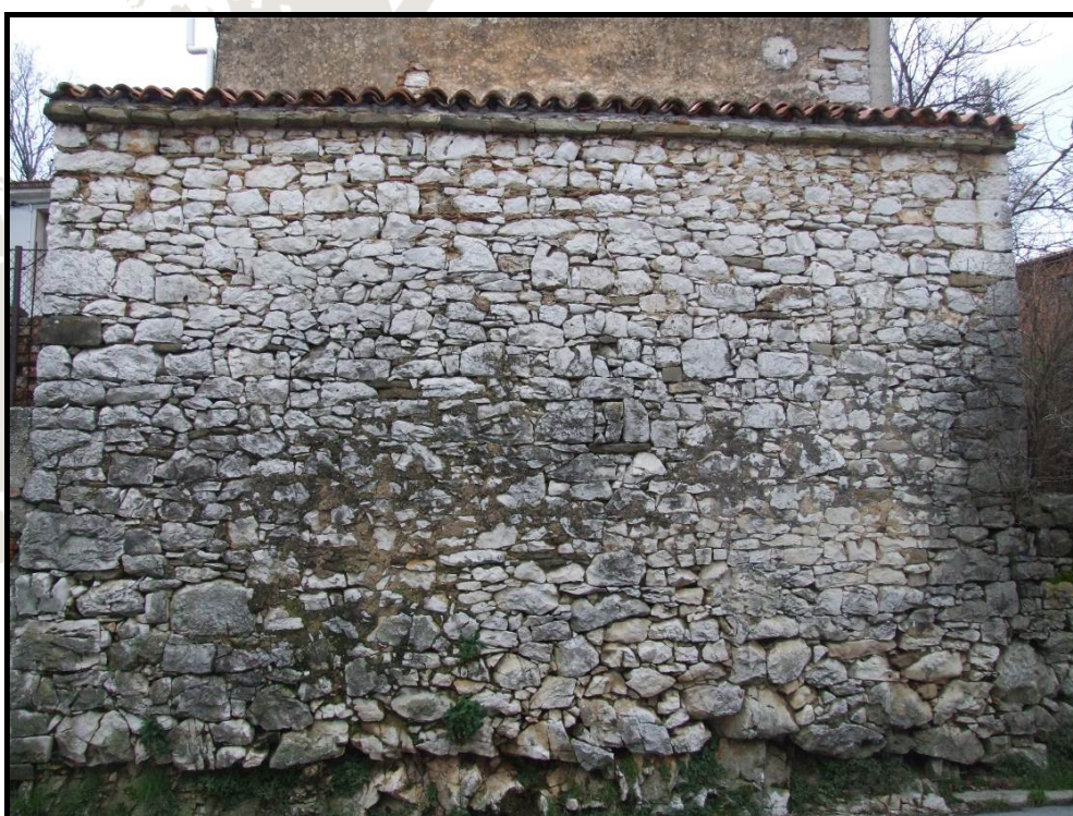
Figure 11. Use of the Alveolinid-numulitid limestone in the village of Grozzana-Gročana actually shows that the stone material might be usable for stonemasonry there.
