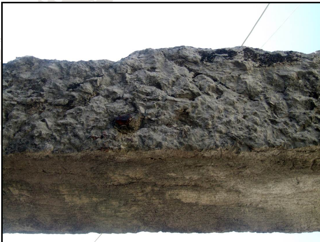
Figure 22. A detail of the rear side of the Architrave from Figure 21 reveals it was originally built-in, and appears here in secondary use.
