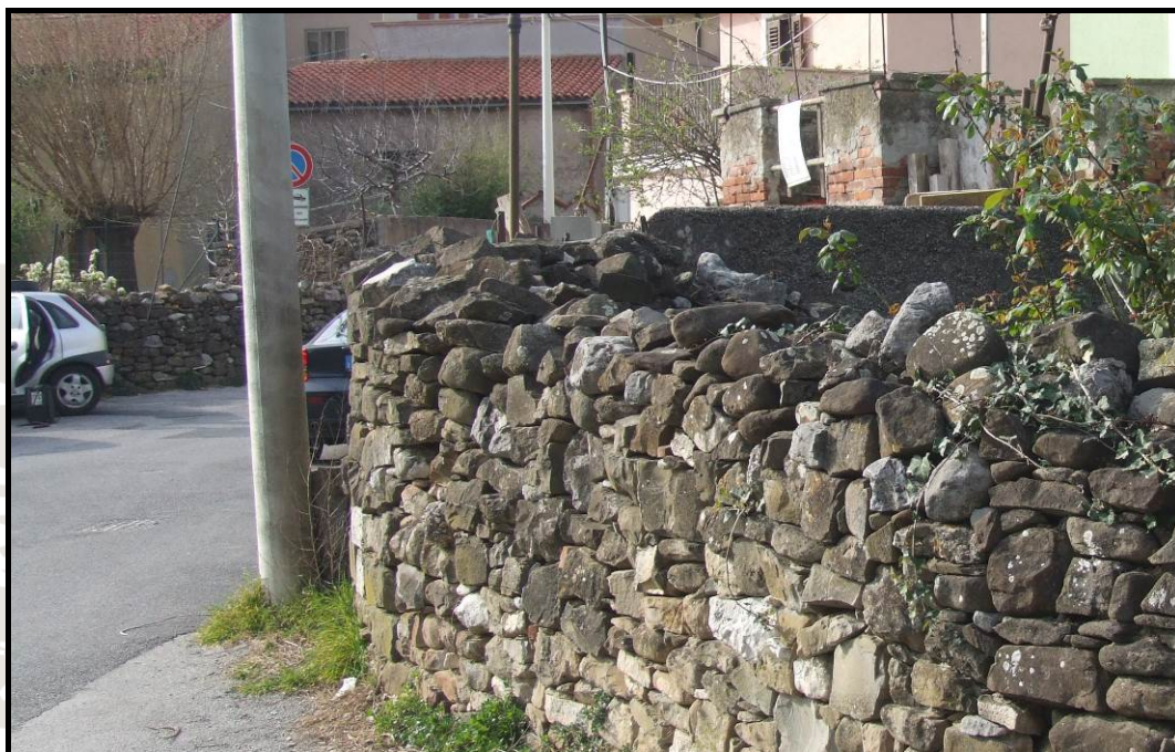
Slika 38. A wall with sandstone pebbles in Bagnoli-Boljunec.
