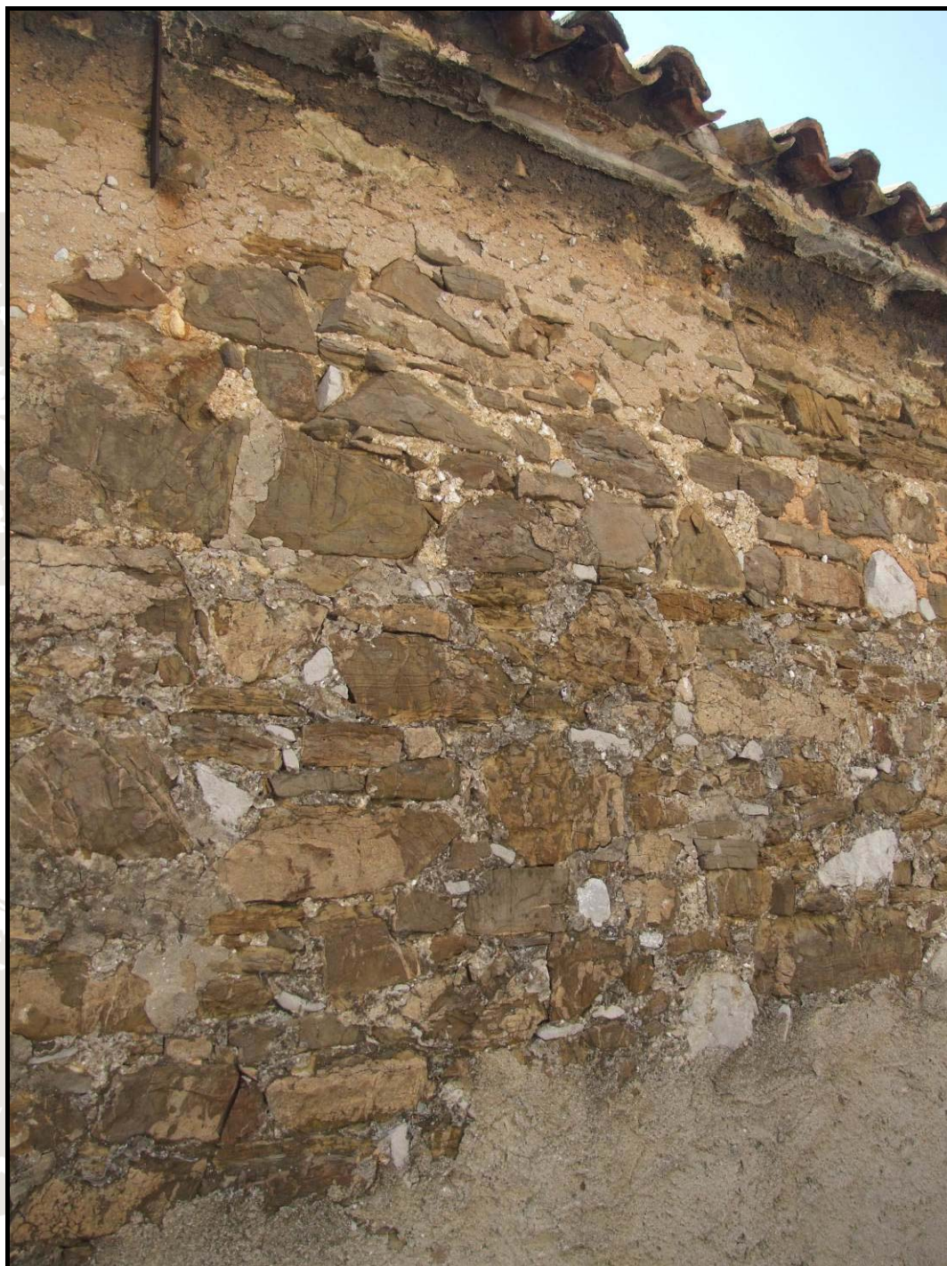
Figure 28. Sandstone blocks with calcite veins are irregular in shape. Occasional blocks of Alveolinid-numulitid limestone are also present (Sant' Antonio in Bosco-Boršt).
