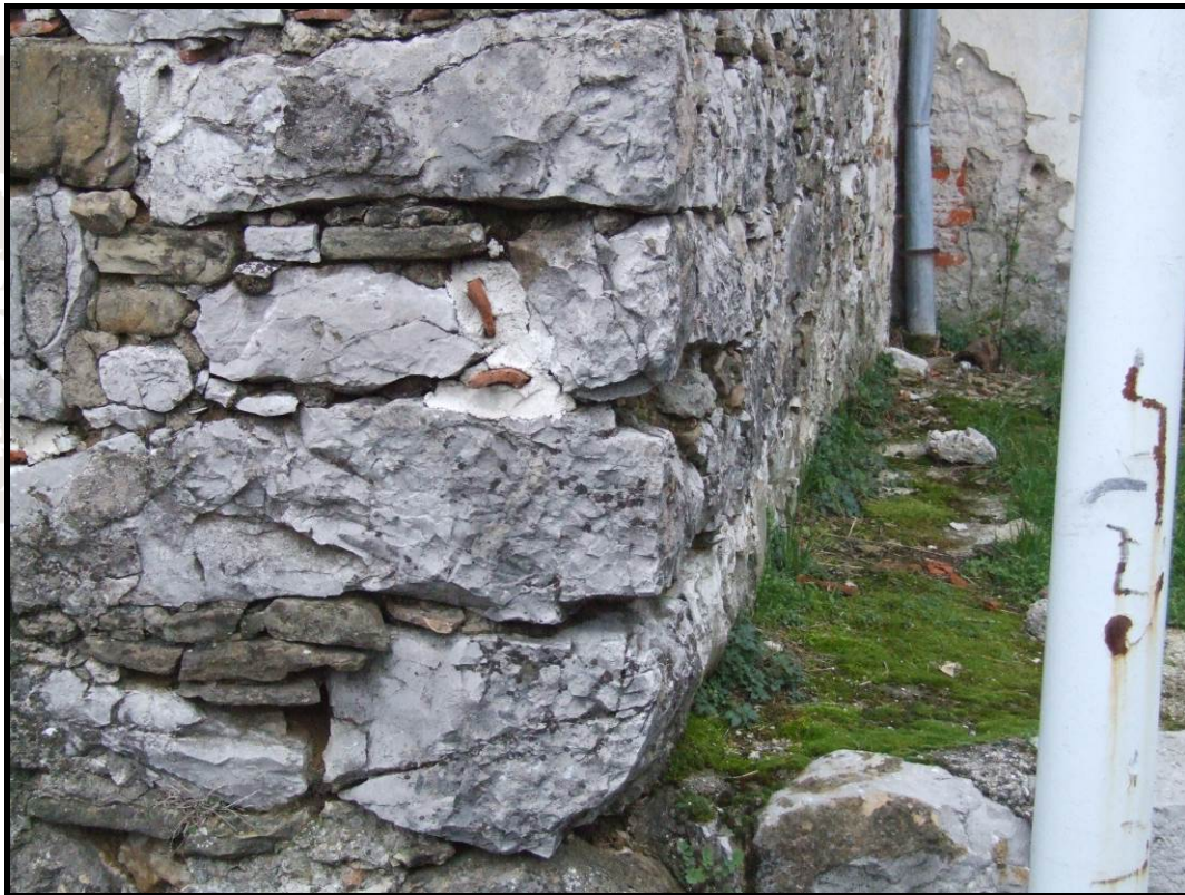
Figure 45. Roughly carved cornerstones made from local limestone at Grozzana-Gročana.
