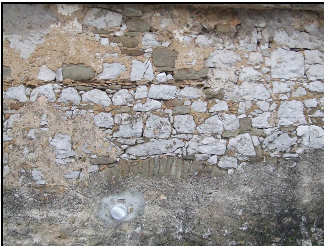
Figure 48. A vault built from flysch sandstone.
