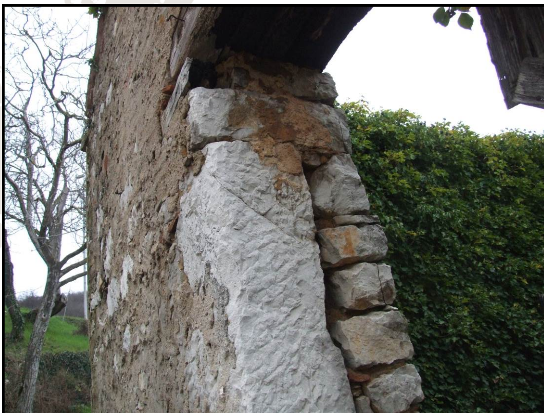
Figure 47. Roughly worked window frame carved from local limestone.
