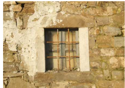
A window frame which reuses side pylons of cretaceous limestone taken from another building
