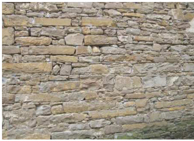
Characteristic construction of peripheral walls from flysch sandstone
