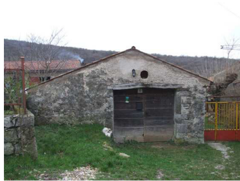
Side framing of a gate built of larger blocks of local limestone and flysch sandstone. The lintel is timber because local stones lack suitable mechanical properties
