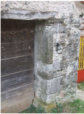
Side framing of a gate built of larger blocks of local limestone and flysch sandstone. The lintel is timber because local stones lack suitable mechanical properties
