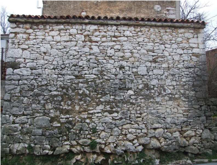
A typical outside wall showing the use of local limestone. Larger and more correctly shaped, roughly treated building stones were used for corners, while the rest of the wall comprises less correctly shaped blocks assembled in horizontal lines. Smaller rocks were used to level the surface. In between are individual blocks of flysch sandstone. They are normally smaller and used mainly for levelling the surface. The wall has traces of rough rendering and inclines to follow the terrain.
