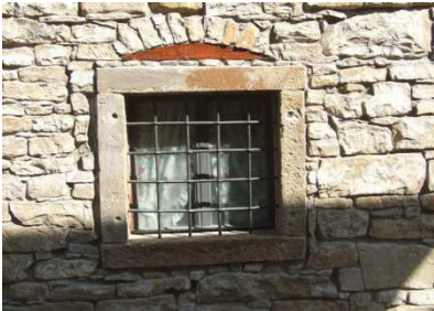
A window reveal of Cretaceous limestone. Above it is a load bearing arch of flysch sandstone, with a timber load bearing element beneath it
