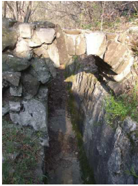
A vault of the Roman aqueduct made from Alveolinid-numulitid limestone and flysch sandstone (left), and of Alveolinid-numulitid limestone exclusively (right).
