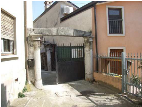
Architrave made of sandstone from the Transitional Beds of Sant' Antonio in Bosco/Boršt.
