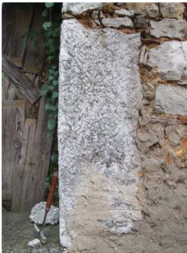
A poor quality stone frame made from local Alveolinid-numulitid limestone (Grozzana/Gročana).
