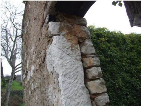
Vertical elements of the window frame (jerte) of local limestone which has been roughly surface treated, in combination with a timber lintel
