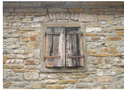
A window frame of flysch sandstone with a load bearing arch also of flysch sandstone. Note the traditional full shutters
