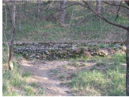
Aqueduct channel made of local Alveolinid-numulitid limestone.
