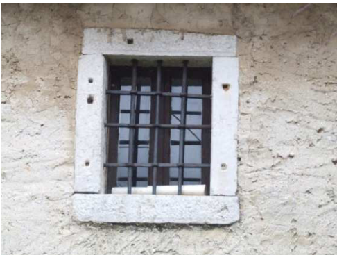
A typical window reveal of Cretaceous limestone from karst quarries
