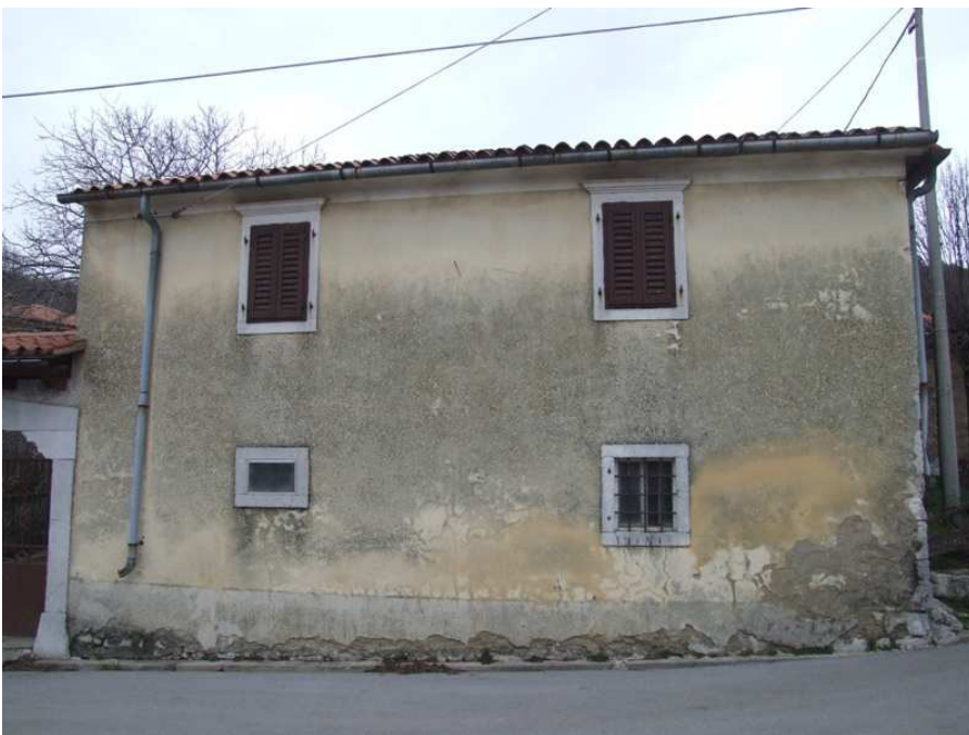
A short semicircular plastered eave over a timber subframe
