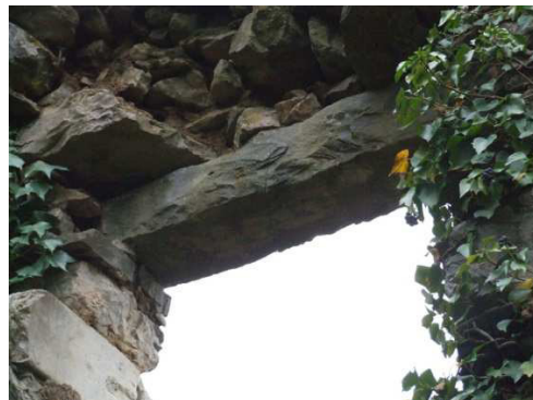
A window lintel of flysch sandstone. The typical cracks visible in the middle manifest pressure overloads.
