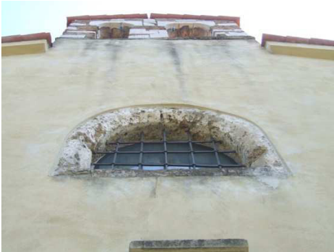
Vaulted window frame made of the local travertine, in the church at Dolina.
