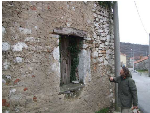
Vertical elements of the window frame (jerte) of local limestone which has been roughly surface treated, in combination with a timber lintel
