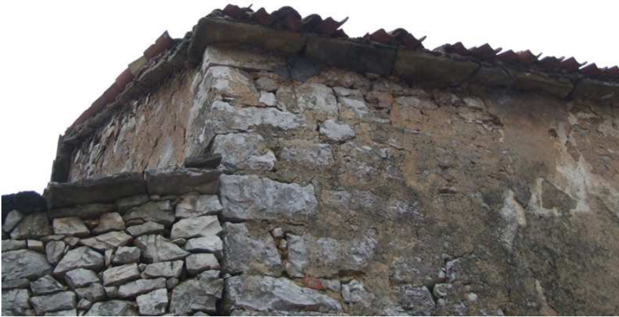
An eave of flysch sandstone grooved roofing tiles and a gabled wall with a row of flysch sandstone grooved roofing flags
