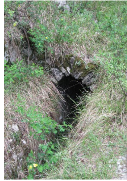
A vault of the Roman aqueduct made from Alveolinid-numulitid limestone and flysch sandstone (left), and of Alveolinid-numulitid limestone exclusively (right).
