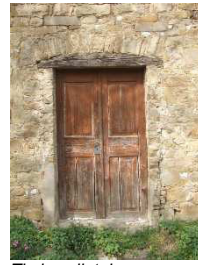
Timber lintel over a gate. Above it is a load bearing stone arch of flysch sandstone building blocks
