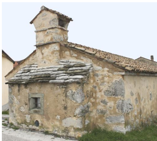
Figure 3. Trebiciano 107, the added kitchen is covered by stone slabs (photo Fabiana Pieri).
